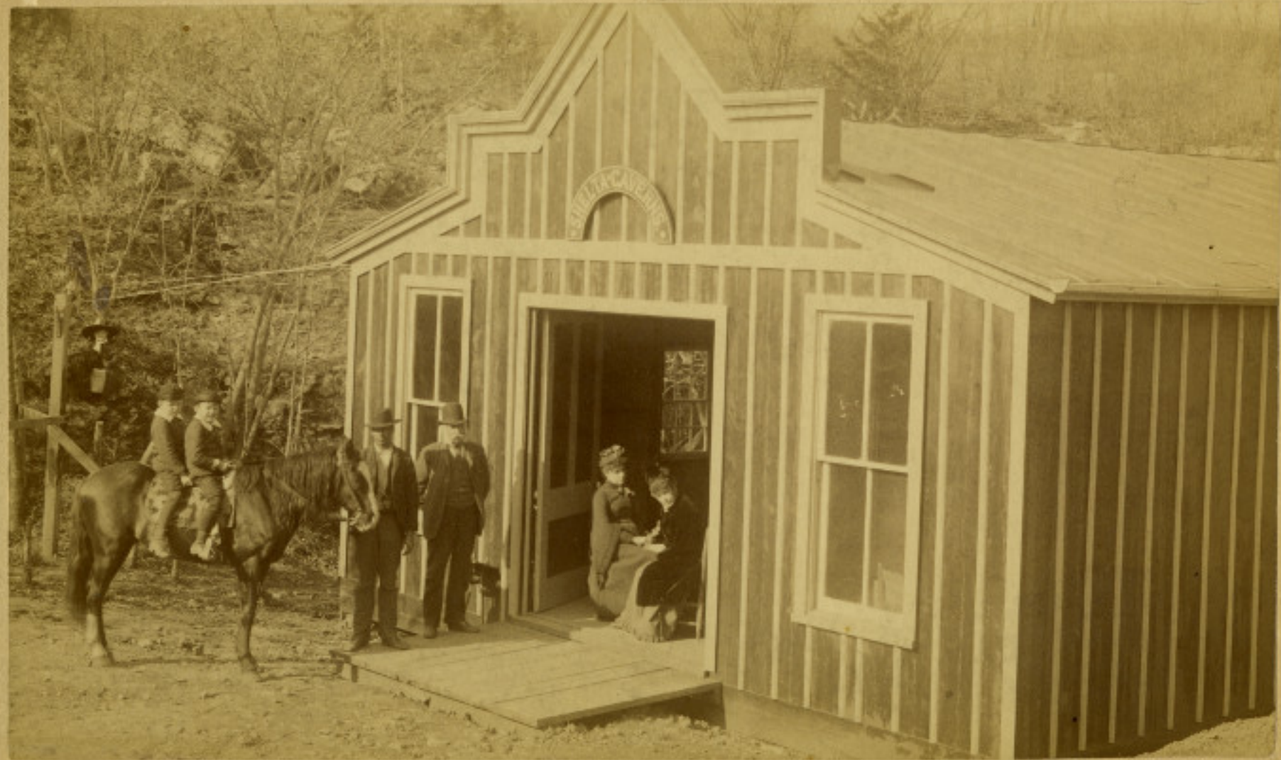
Entrance to Shelta Pavilion
