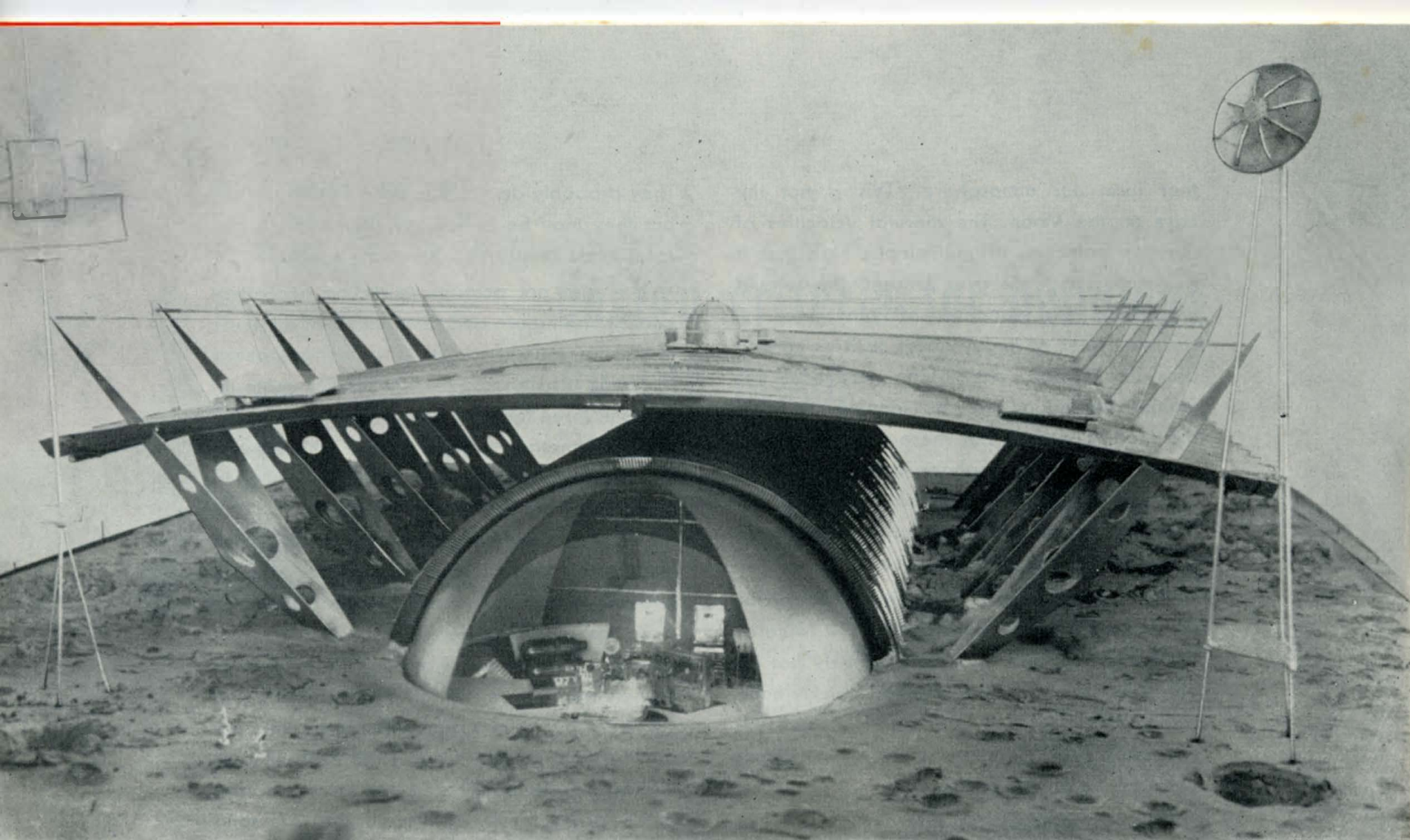
Scale model of a Moon building designed and built by the Wonder Building Corporation of America, as a permanent structure for our Moon explorers. The plastic bubble-type observatory in the foreground is protected from ultraviolet radiation by sliding metal doors. The overhead structure is a meteorite shield to protect the building proper. The dome in the center of the barrier is a traffic control tower. The proposed building would be 340 feet long, 160 feet wide, and 65 feet high.
