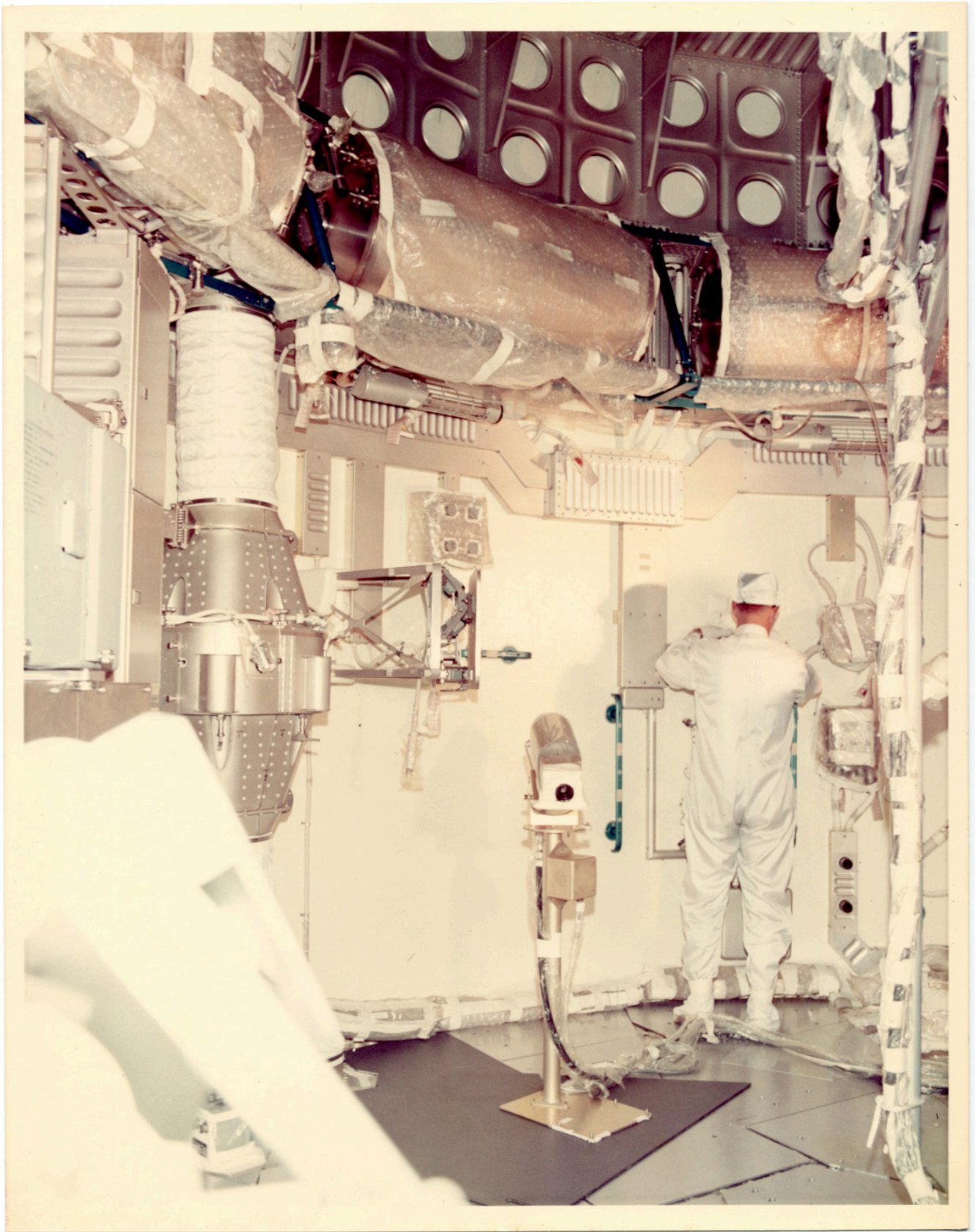
There is a still caption on the back which reads: "INTERIOR VIEW OF UPPER LEVEL. OWS NO. 1."
