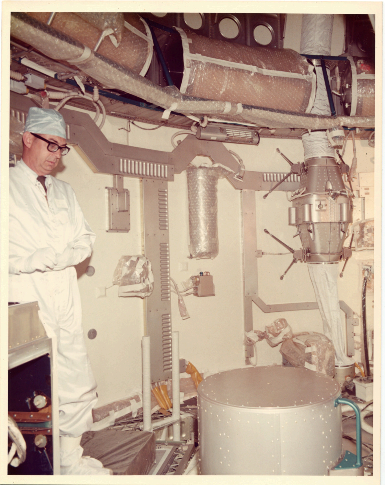
There is a still caption on the back which reads: "INTERIOR VIEW OF UPPER LEVEL OWS NO. 1."
