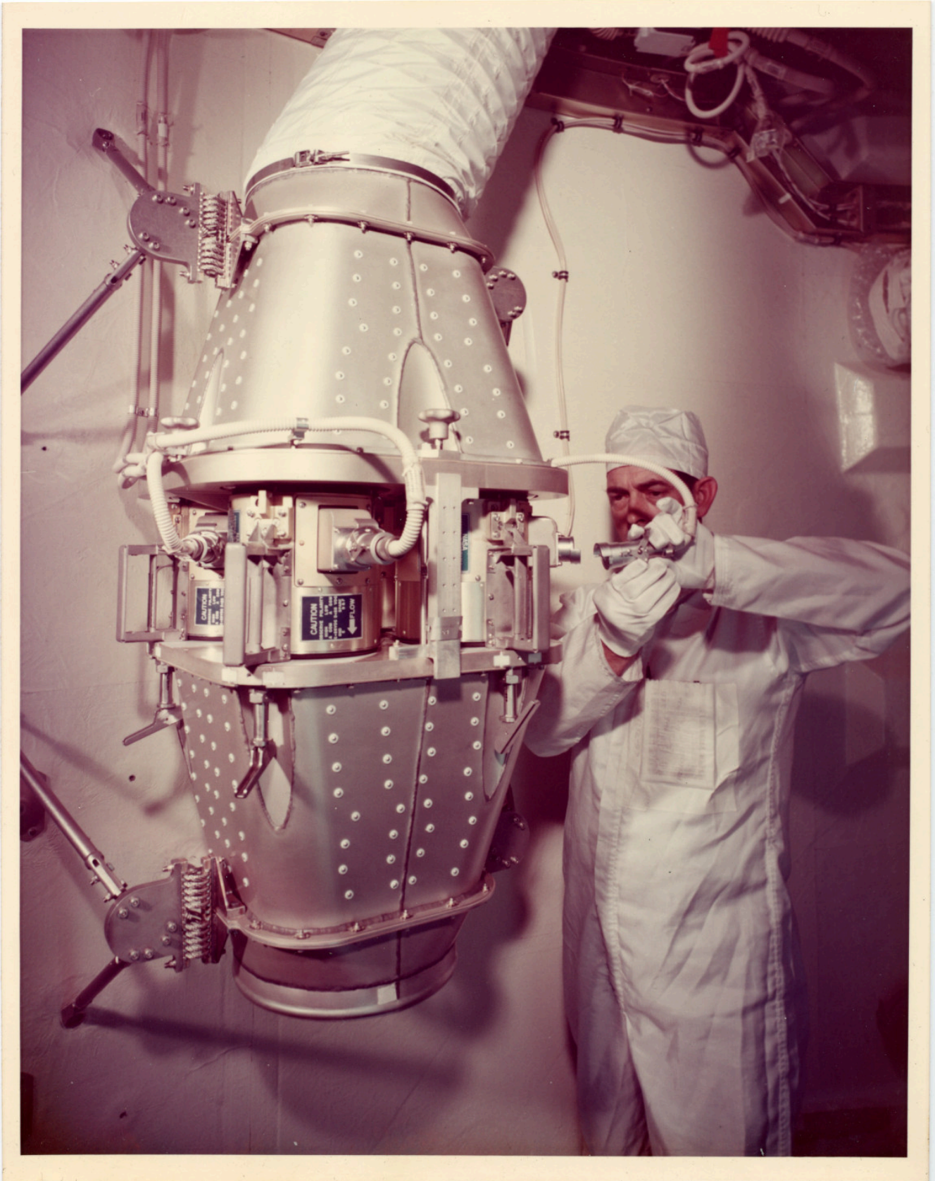
There is a still caption on the back which reads: "CONNECTING POWER LEAD TO FAN CLUSTER. OWS NO. 1."
