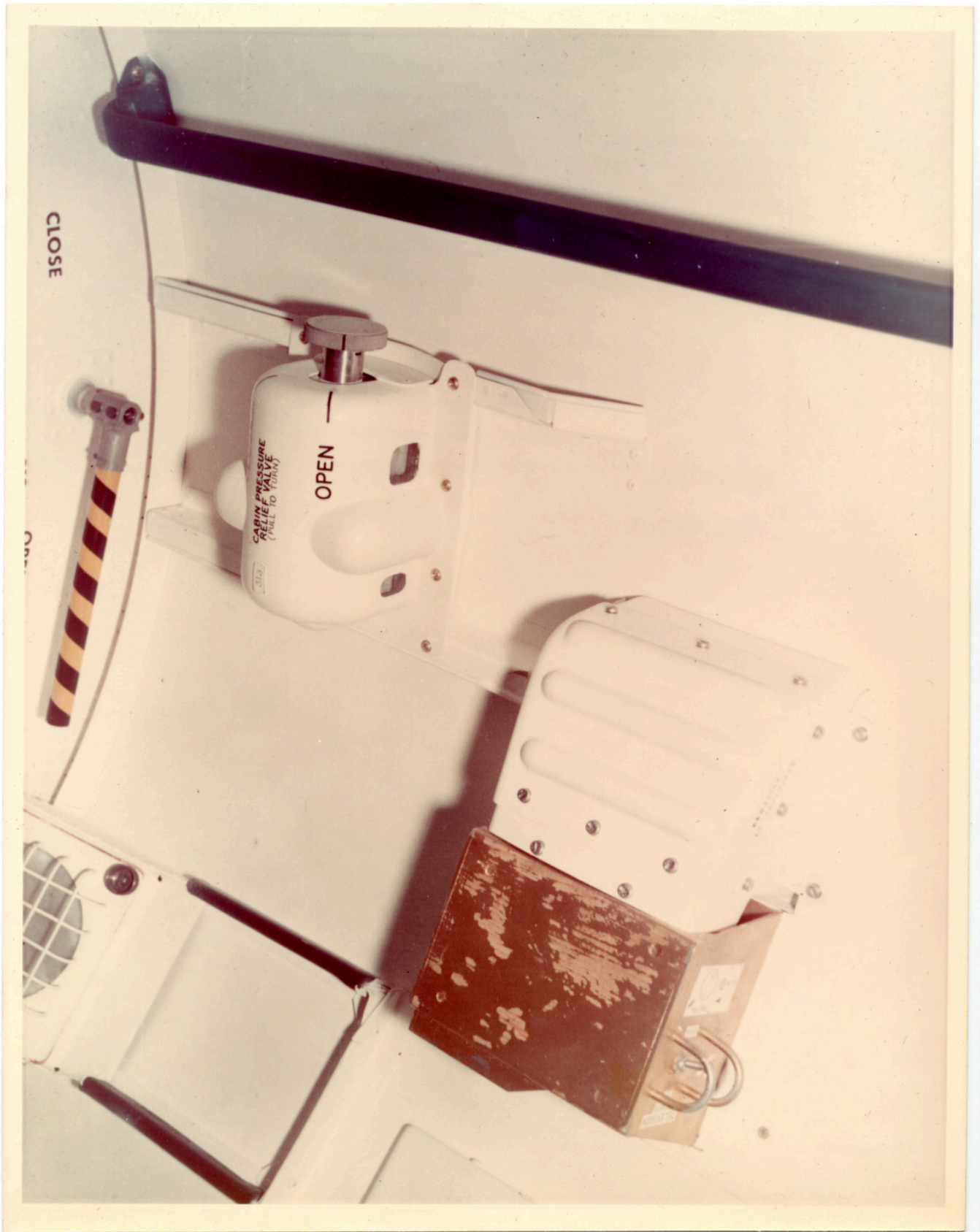
There is a still caption on the back which reads: "NASA TRAINER - LOCK COMPARTMENT - CLOSEUP OF TV STATION. PRESSURE RELIEF VALVE 313. AND 20 WATT TUNNEL LIGHT NASA-1619"
