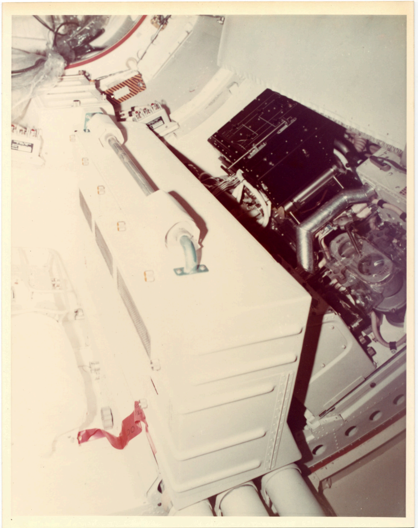
There is a still caption on the back which reads: "Airlock Zone 1 internal section of STS between +Y and -Z axis showing tunnel interface near spare condensate tank module AM circulation fans and Mol Sieve "B" Mdac Input for month of June."
