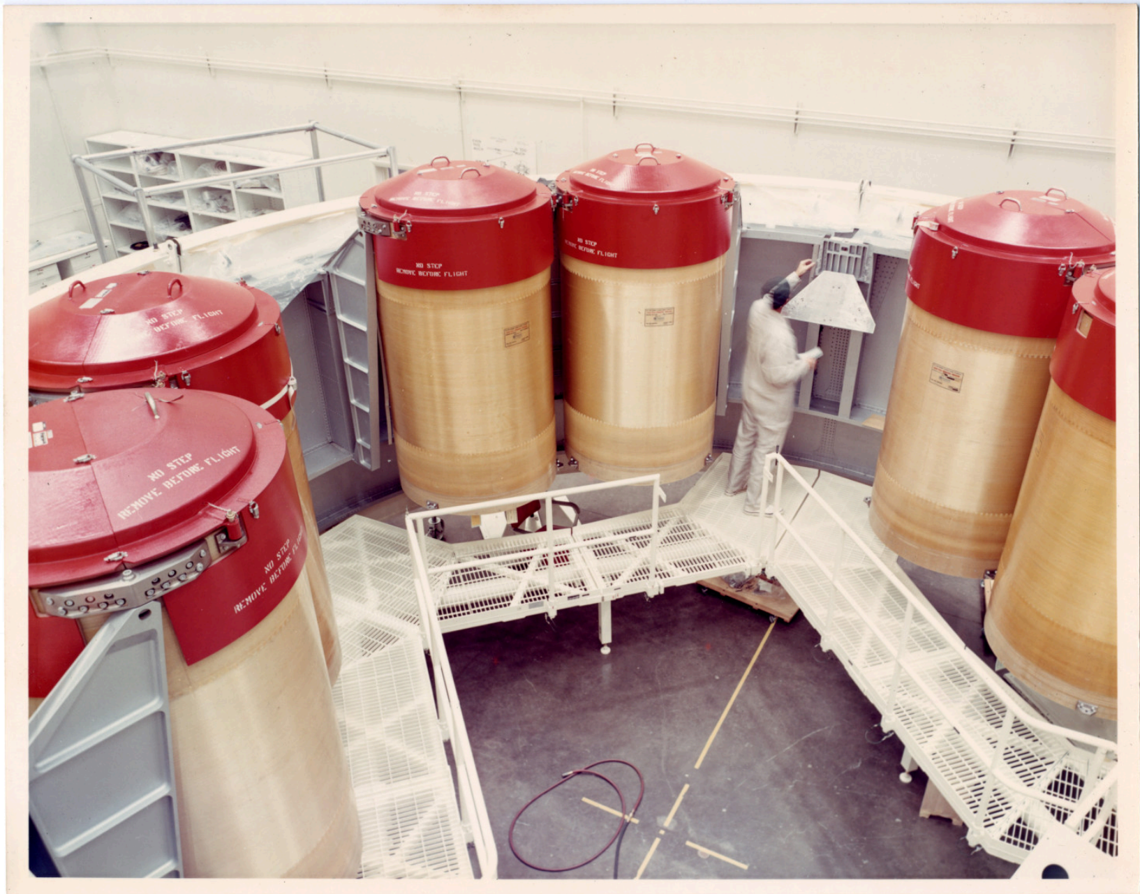
There is a still caption on the back which reads: "AIRLOCK FLIGHT ARTICLE NO. 1 FAS IN CLEAN ROOM. INSTALLATION OF OXYGEN TANKS."
