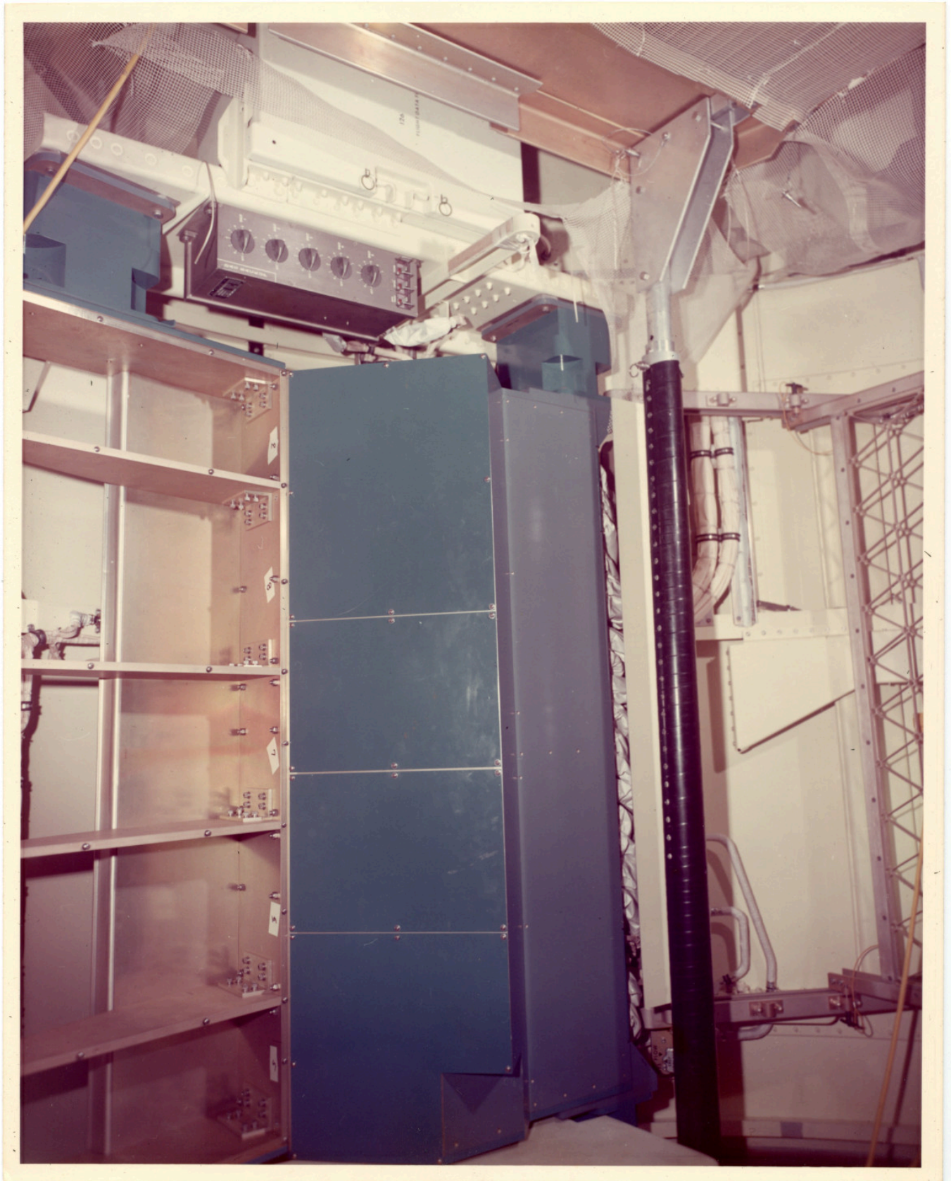
There is a still caption on the back which reads: "MDA Backup Article Final wire installation for ATM/C&D Console end digital address system backup. MDAC Input for month of June"
