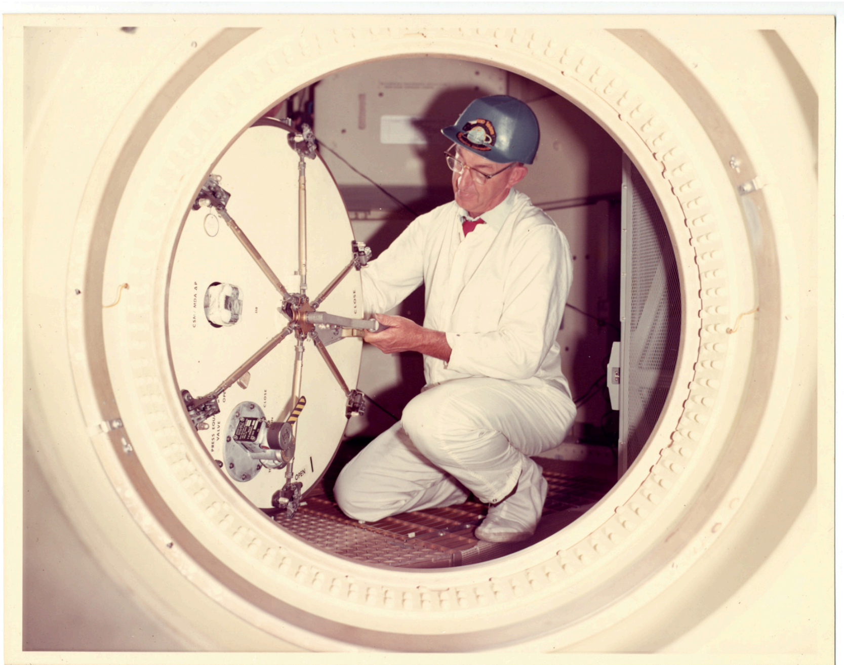
There is a still caption on the back which reads: "OPERATING AXIAL DOCKING PORT DOOR DURING CLOSURE TEST. MDA BACKUP ARTICLE. MDAC INPUT FOR JULY."
