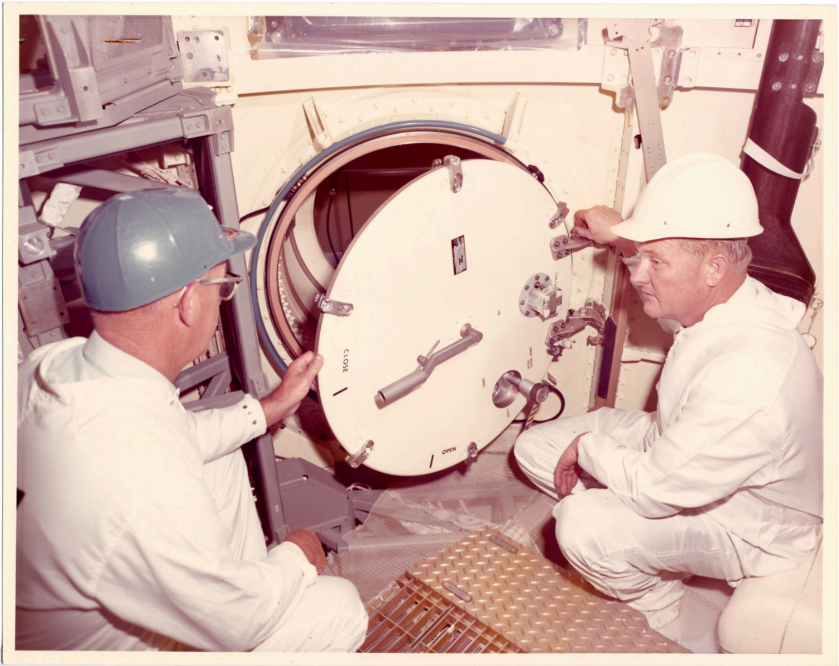
There is a still caption on the back which reads: "INSTALLATION OF AXIAL DOCKING PORT HATCH DOOR DURING TEST. MDA BACKUP ARTICLE. MDAC INPUT FOR JULY."
