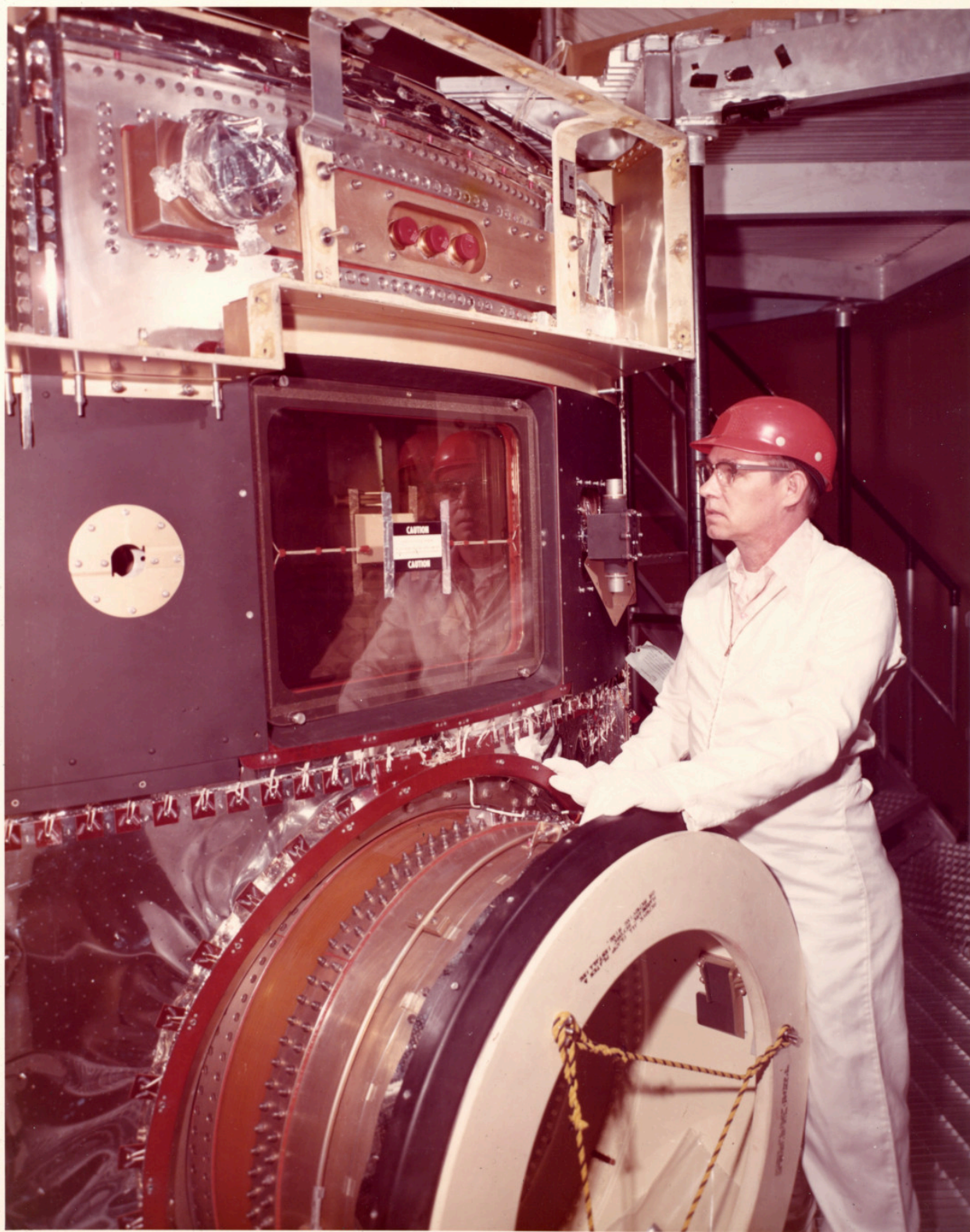
There is a still caption on the back which reads: "MDA BACKUP ARTICLE. CHECKING METEOROID SHIELD INSTALLATION IN AREA OF S190 WINDOW AND RADIAL PORT"
