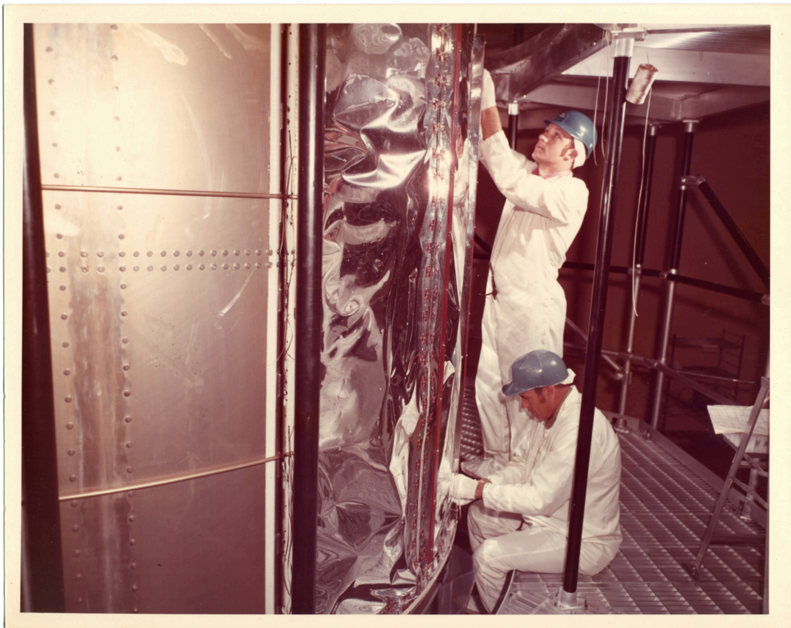
There is a still caption on the back which reads: "MDA BACKUP ARTICLE SHOWING INSTALLATION OF INSULATION BLANKETS"
