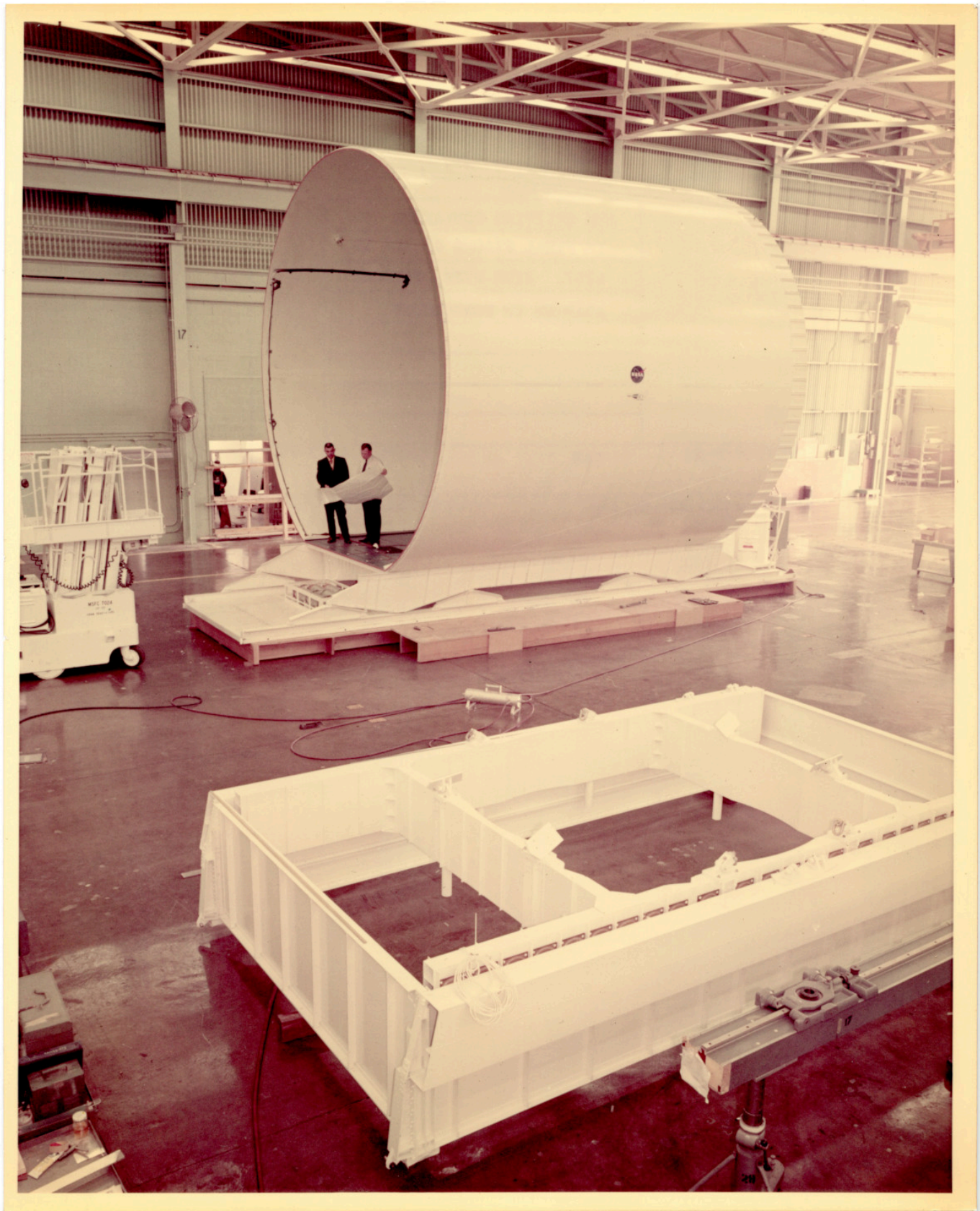
There is a Still Caption on the back that reads, "ATM SHIPPING CONTAINER IN FINAL STAGES OF FAB IN 4707. SIDE VIEW, PAYLOAD ADAPTER IN FOREGROUND."
