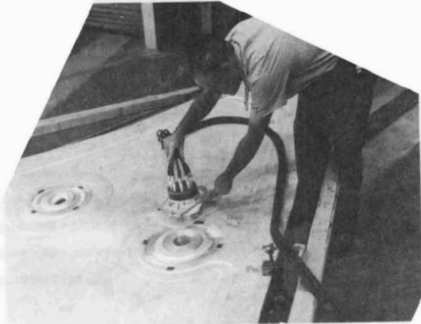
FIGURE 1-8. MAGNETIC HAMMER
