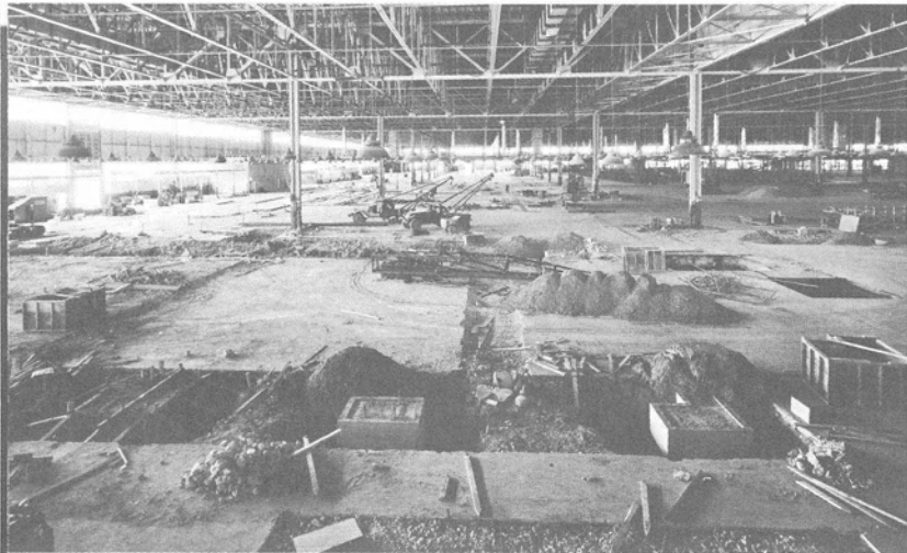
The manufacturing building during renovation
