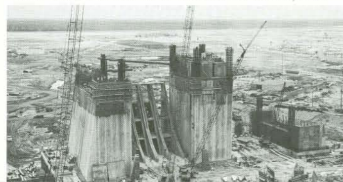
Photo shows S-IC test-stand construction October, 1965.
