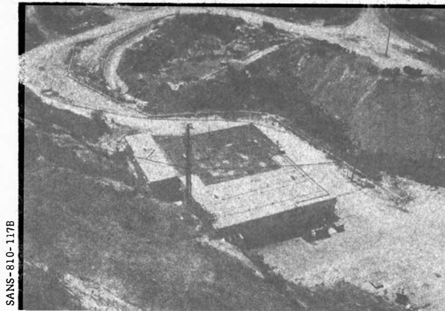
Figure IV-17. Closeup of Control Center
