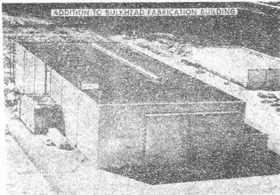
Figure IV-5. Addition to Bulkhead Fabrication Building
