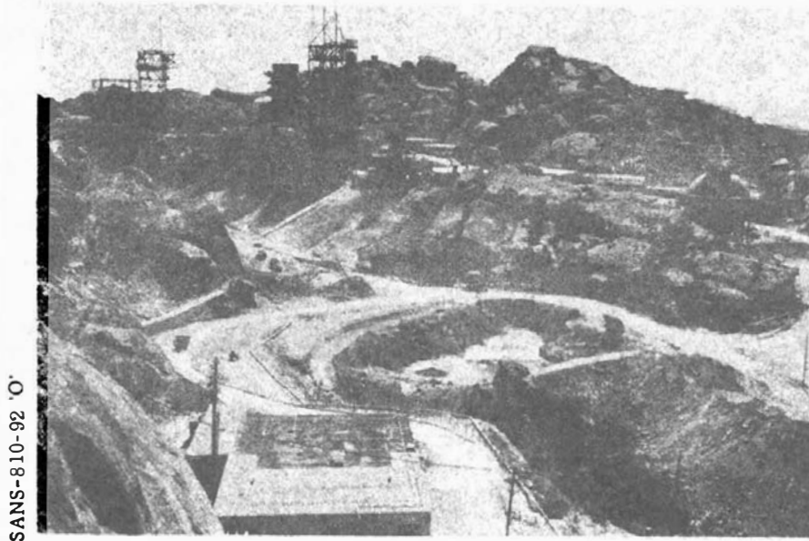
Figure IV-16. SSFL Control Center
