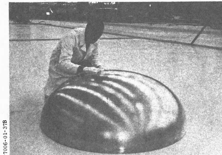
Figure 16. Ellipsoidal Model Bulkhead, Exterior View
