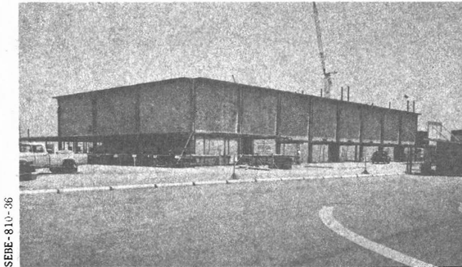
Figure 77. Service Building Construction as of 30 June 1963
