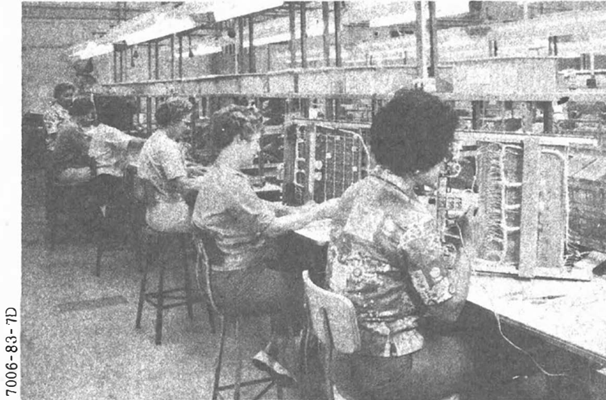
Figure 44. Assembly Operation of the Logic Drawers for the Automatic Rack of the Breadboard Test Set
