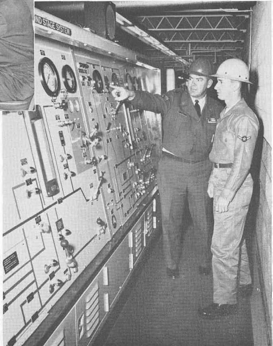
T/Sgt. Billy E. Cook, Atlas missile hydraulics instructor, explains the operation of complex ground support equipment to A3C John McCoy.
