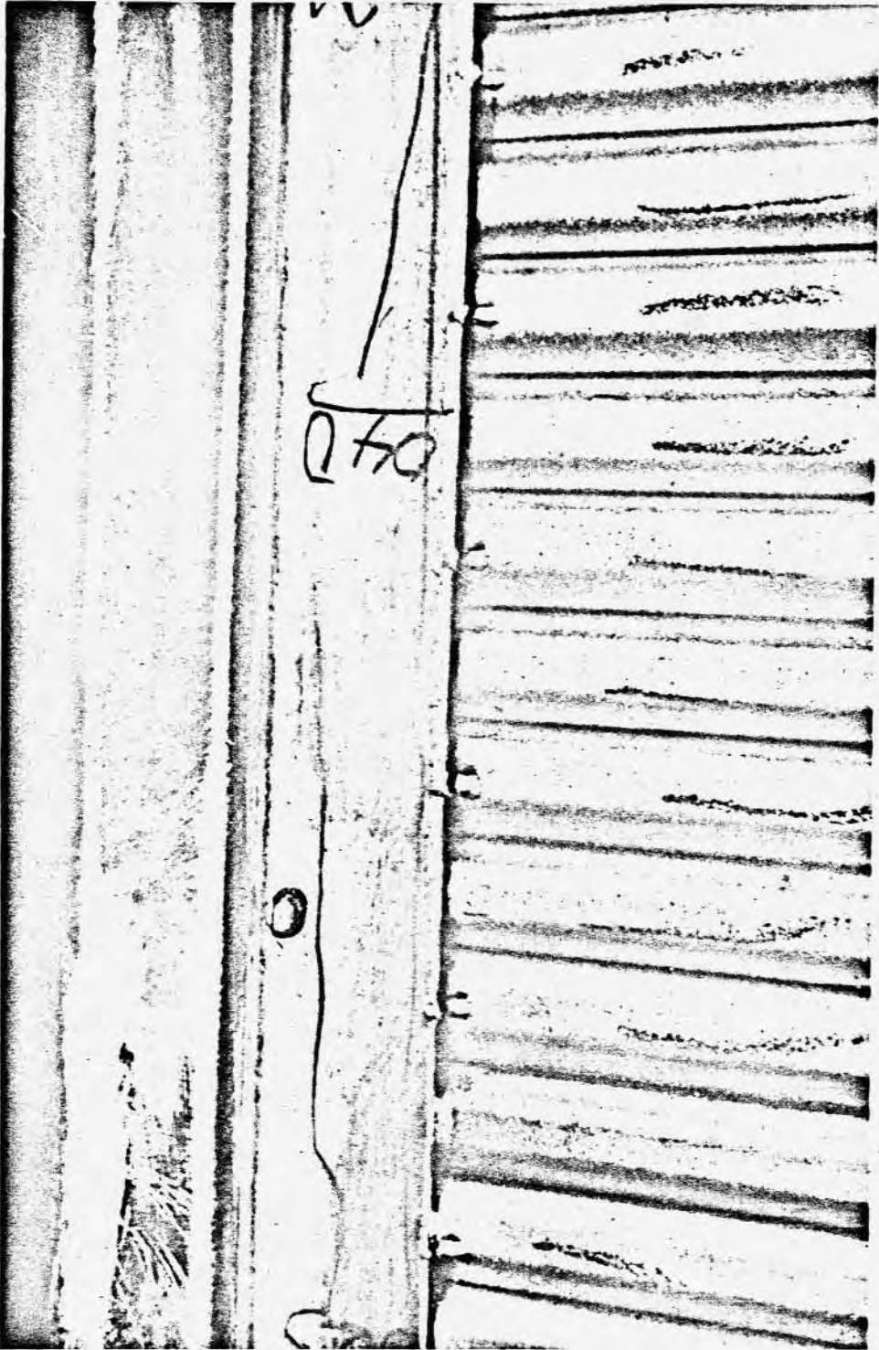
Figure 14. Tube-To-Band Tack Welds Pulled Loose
