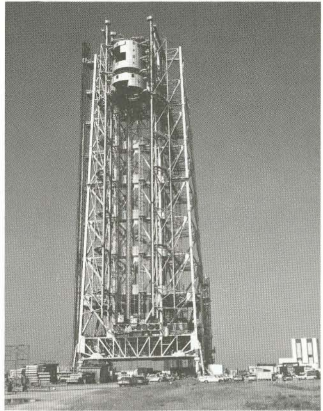
Mobile Service Structure at its parking area
