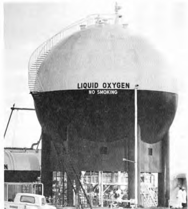
Liquid oxygen service facility
