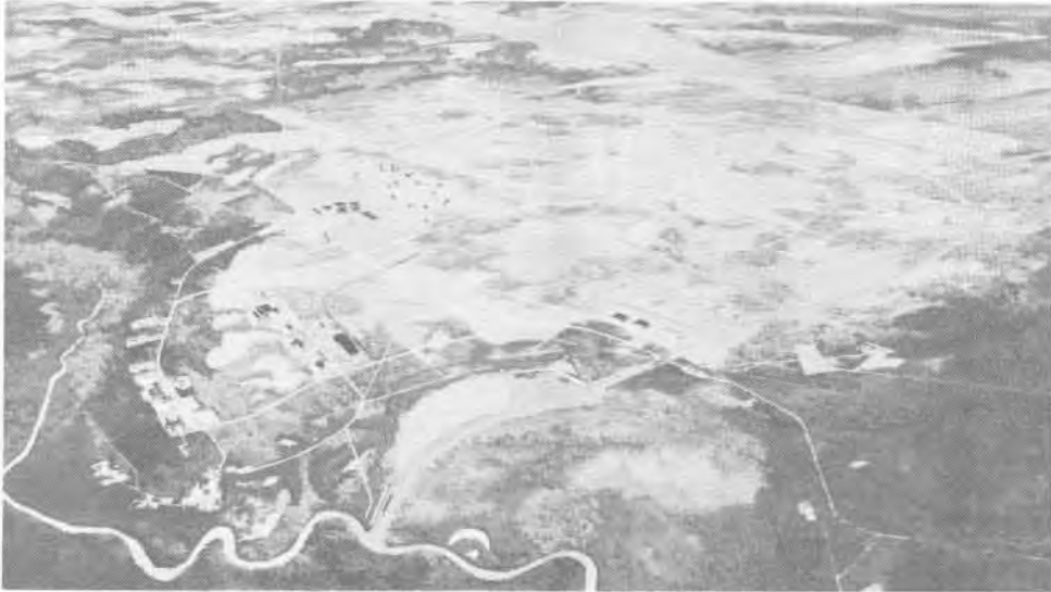
FIGURE 111. MISSISSIPPI TEST FACILITY
