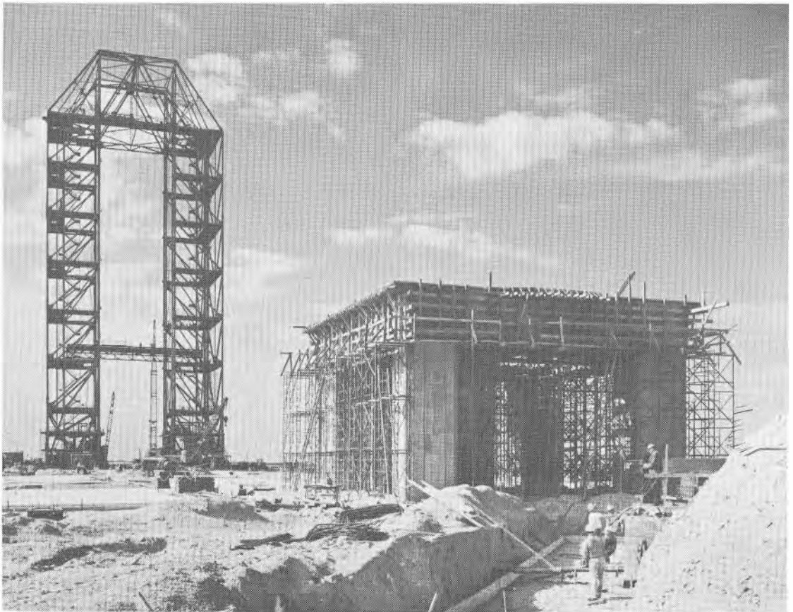
FIGURE 26. CONSTRUCTION OF SERVICE TOWER AND PEDESTAL
