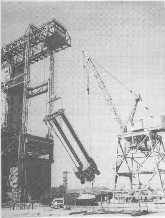
FIGURE 64. INSTALLATION OF SA-T2 ON STATIC TEST STAND
