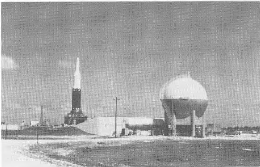
FIGURE 94. SA-2 ERECTED ON LAUNCH PEDESTAL
