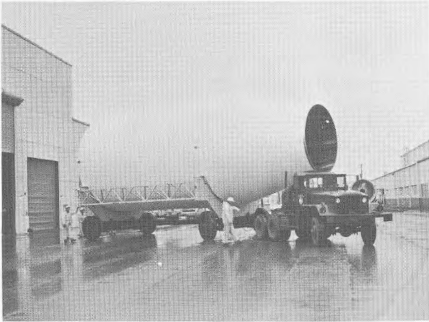
FIGURE 34. MOVEMENT OF DUMMY S-IV STAGE TO CHECKOUT
