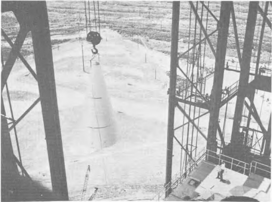
FIGURE 80. PAYLOAD BODY ERECTION INTO SERVICE STRUCTURE
