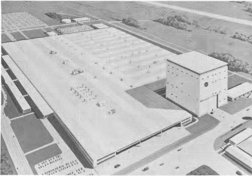
FIGURE 112. VERTICAL ASSEMBLY BUILDING AT MICHLOUD
