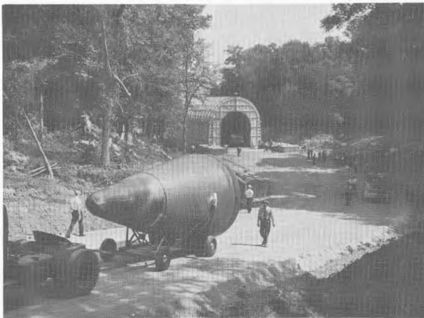
FIGURE 74. PAYLOAD MOVEMENT AROUND WHEELER DAM
