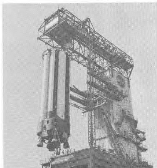
FIGURE 48. POSITIONING FLIGHT BOOSTER IN TEST STAND
