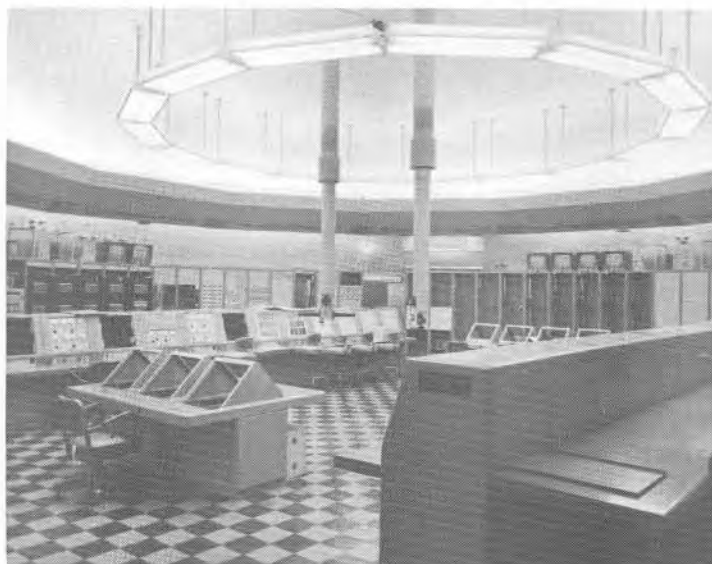
FIGURE 59. LAUNCH COMPLEX 34, BLOCKHOUSE INTERIOR
