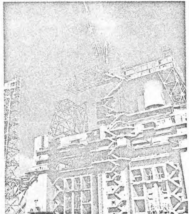
Figure 3-5 Erection of West Pier (B-1) Upper Steel Work
