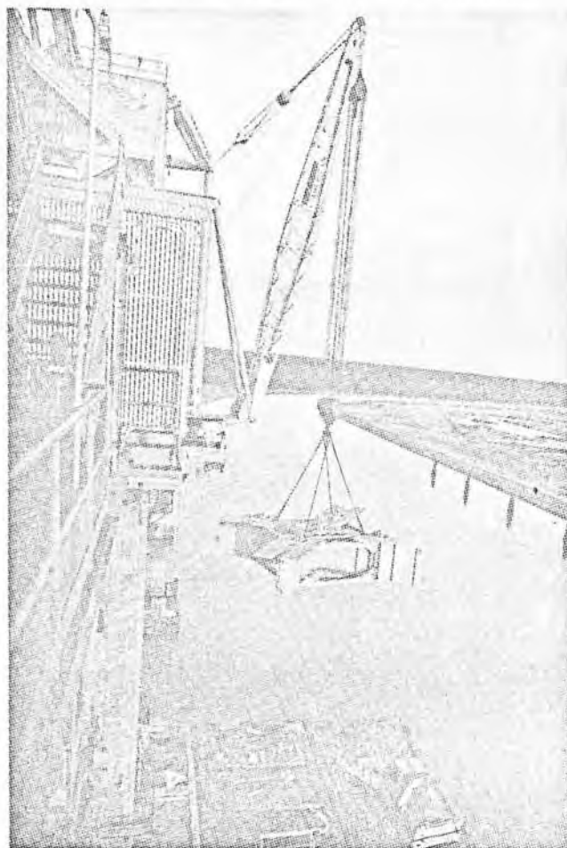
Figure 3-7 "Spider" Being Hoisted Into Test Stand
