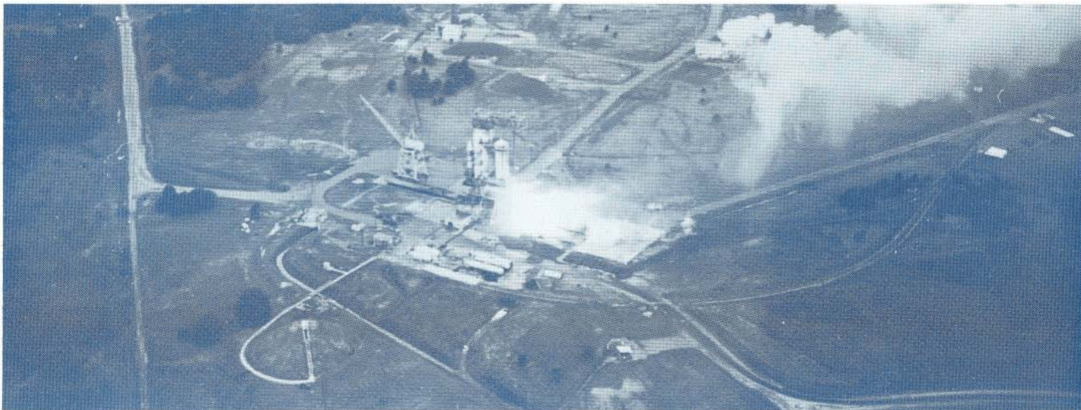
The static test of an early S-I stage as seen from an observation plane. The flame of the exhaust is deflected by a water-cooled scoop at the base of the tower.
