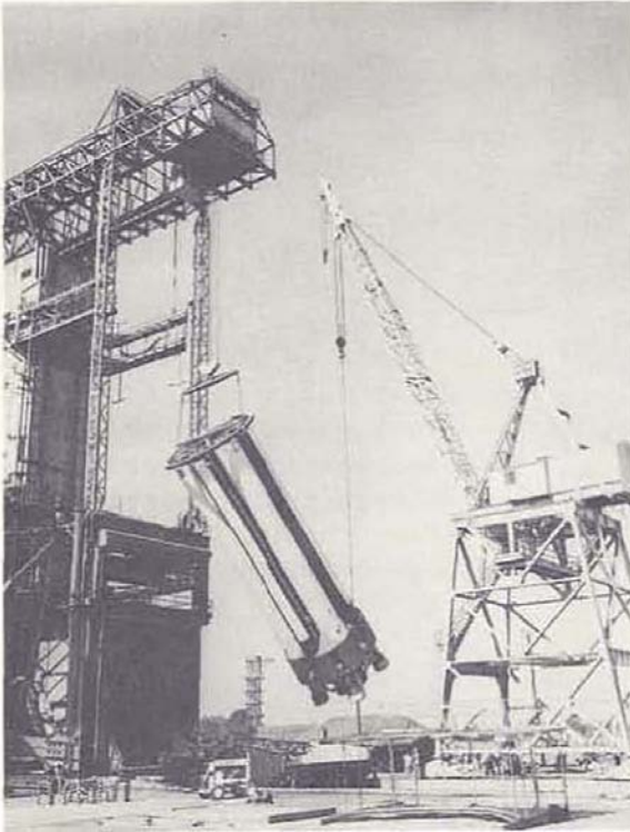
FIGURE 64. INSTALLATION OF SA-T2 ON STATIC TEST STAND
