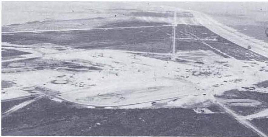
FIGURE 97. CONSTRUCTION OF LAUNCH COMPLEX 37
