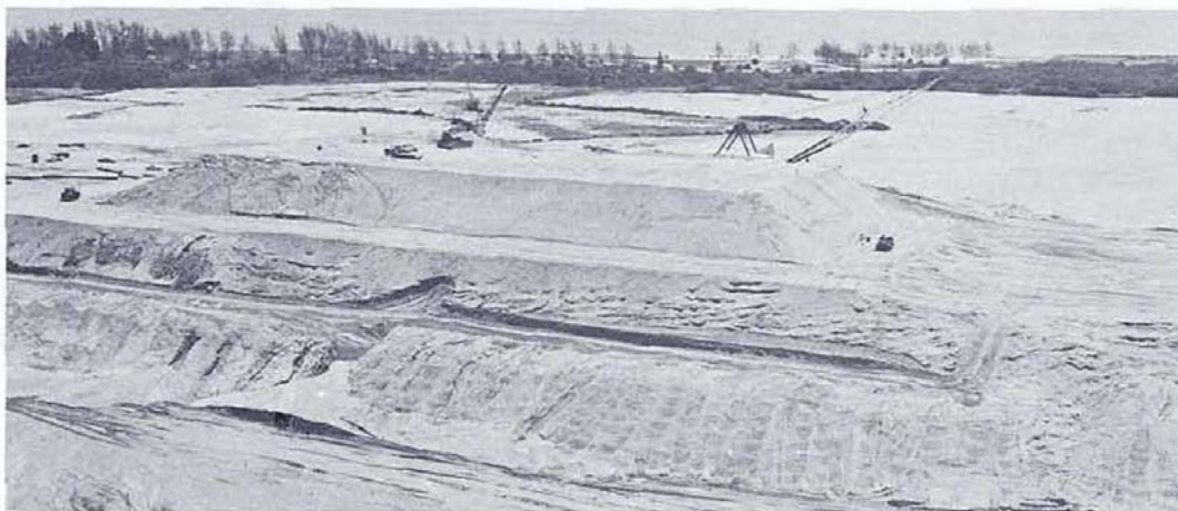
FIGURE 148. CONSTRUCTION AT LAUNCH COMPLEX 39
