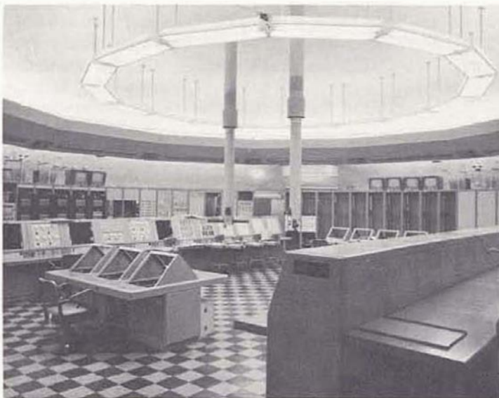
FIGURE 59. LAUNCH COMPLEX 34, BLOCKHOUSE INTERIOR
