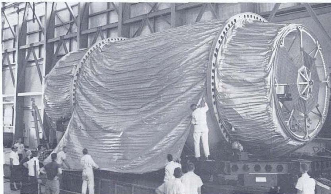
FIGURE 121. S-IV DYNAMIC/FACILITIES AT CAPE CANAVERAL
