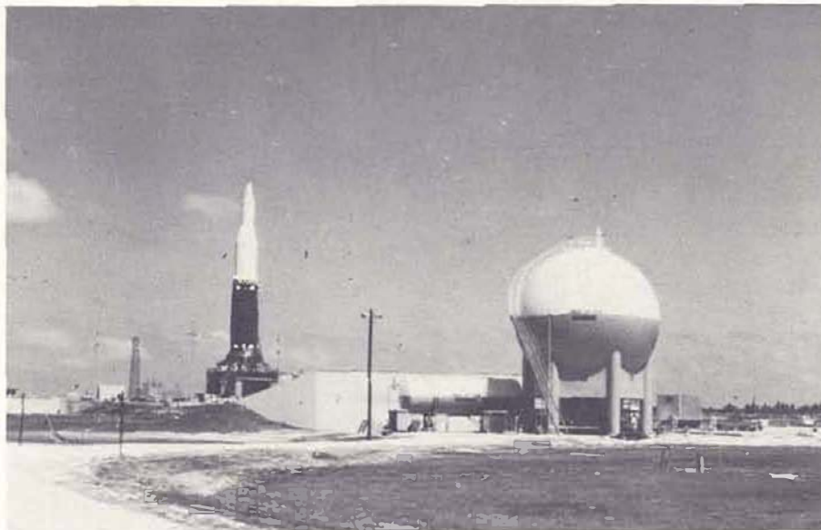
FIGURE 94. SA-2 ERECTED ON LAUNCH PEDESTAL
