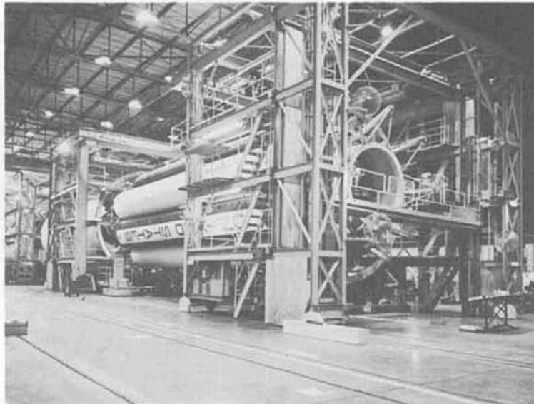
FIGURE 22. STRUCTURAL FABRICATION OF SA-1 BOOSTER
