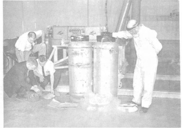
Figure III-12 - Shrink Fitting--Temperature Inspection During Freezing of Bulkhead Fitting Prior to Welding Operation
