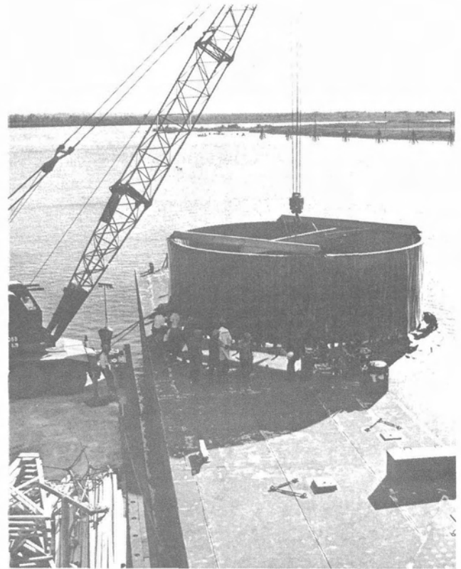
Figure IX-2 - The Half Intertank is Carefully Loaded on the Barge at the Dock and Secured by Boeing Mechanics
