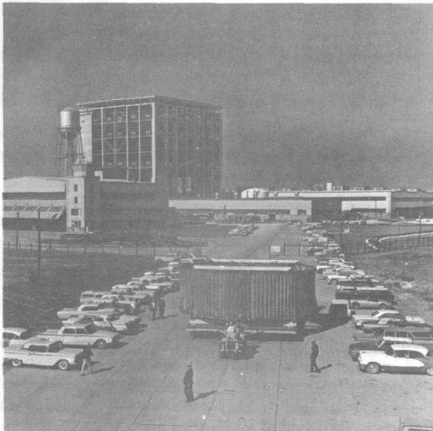
Figure IX-1 - The Michoud Plant and the Partially Completed Vertical Assembly Building are a Backdrop for the One-Half Intertank Being Towed to the Slip for Shipment to MSFC
