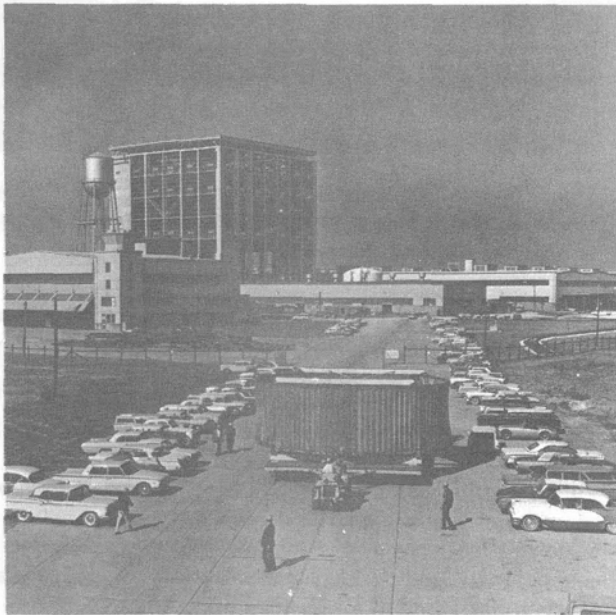
Figure IX-1 - The Michoud Plant and the Partially Completed Vertical Assembly Building are a Backdrop for the One-Half Intertank Being Towed to the Slip for Shipment to MSFC
