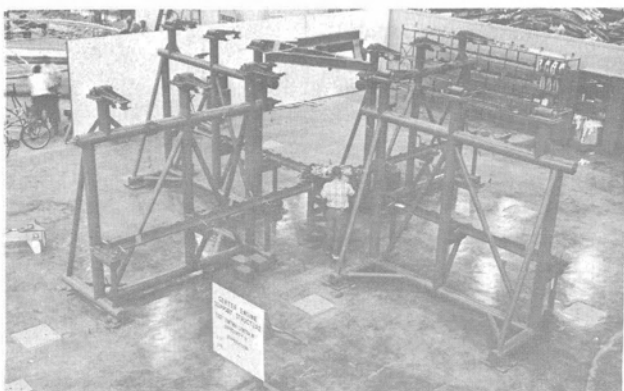
Figure III-3 - Assembly Fixture Used For the Center-Engine Support Nears Completion.
