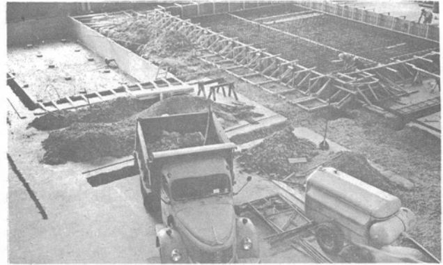
Figure IV-3 - Construction Progress of Permanent Quality Evaluation Laboratories at Michoud
