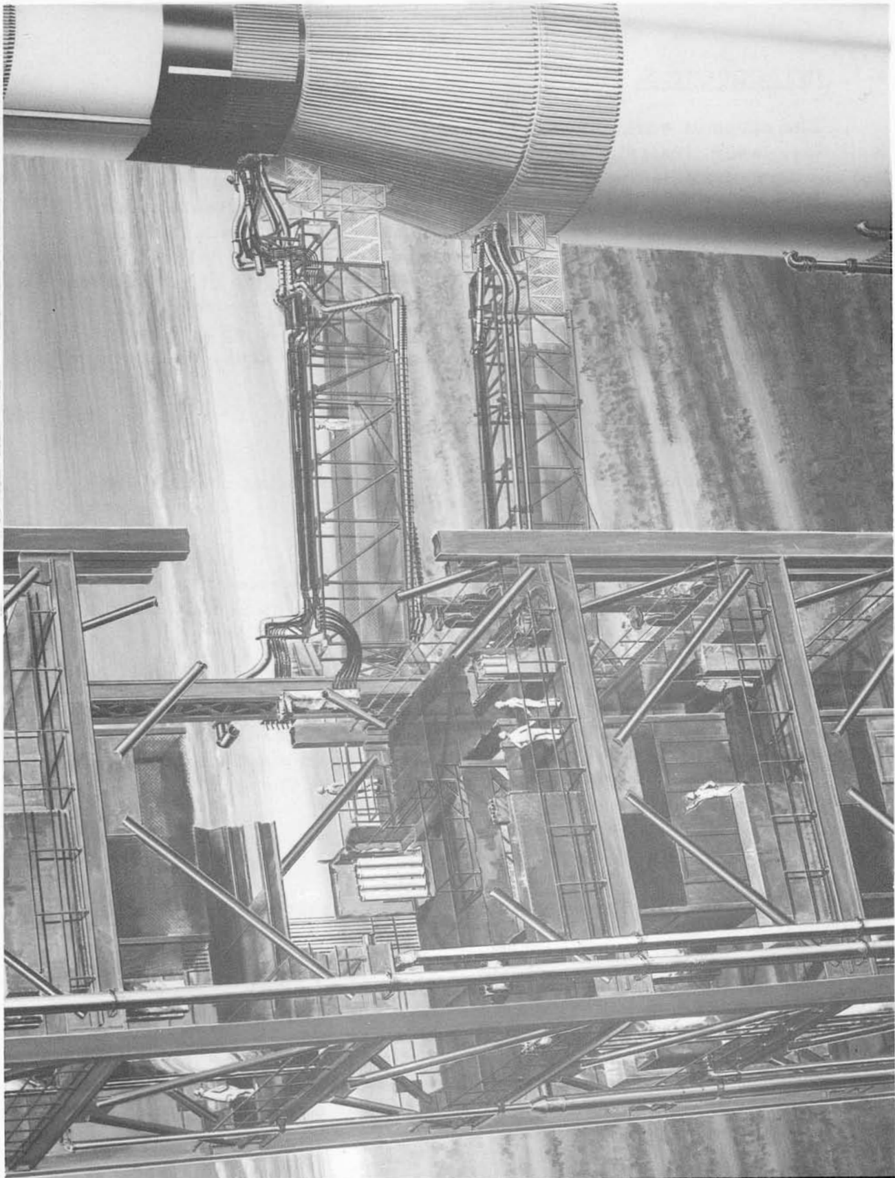
Figure 1-1. S-IVB AFT and S-II FWD Service Arms and Associated Equipment
