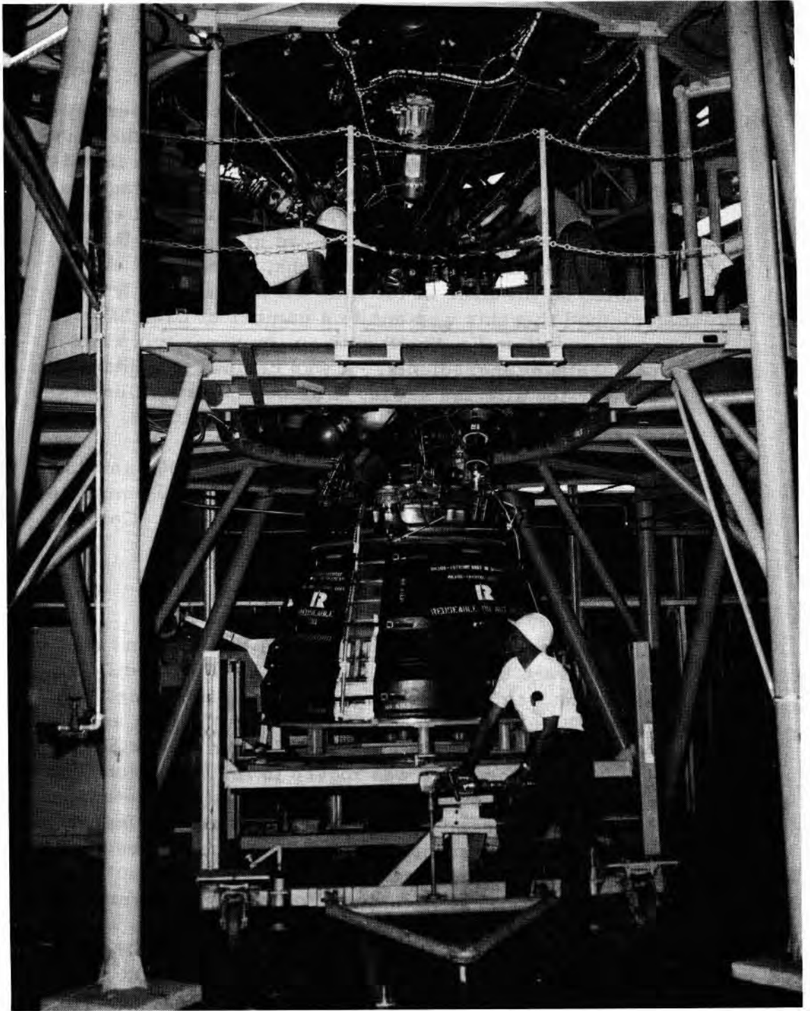
Figure 13. J-2 Engine Installed In The S-IVB-506.
