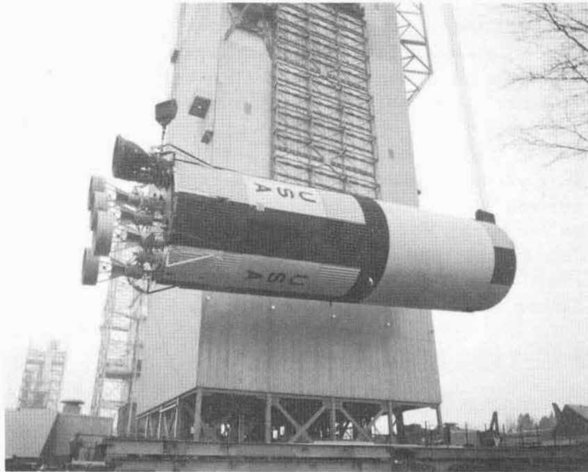
Figure 1 - S-IC-D Being Raised Into MSFC Dynamic Test Stand
