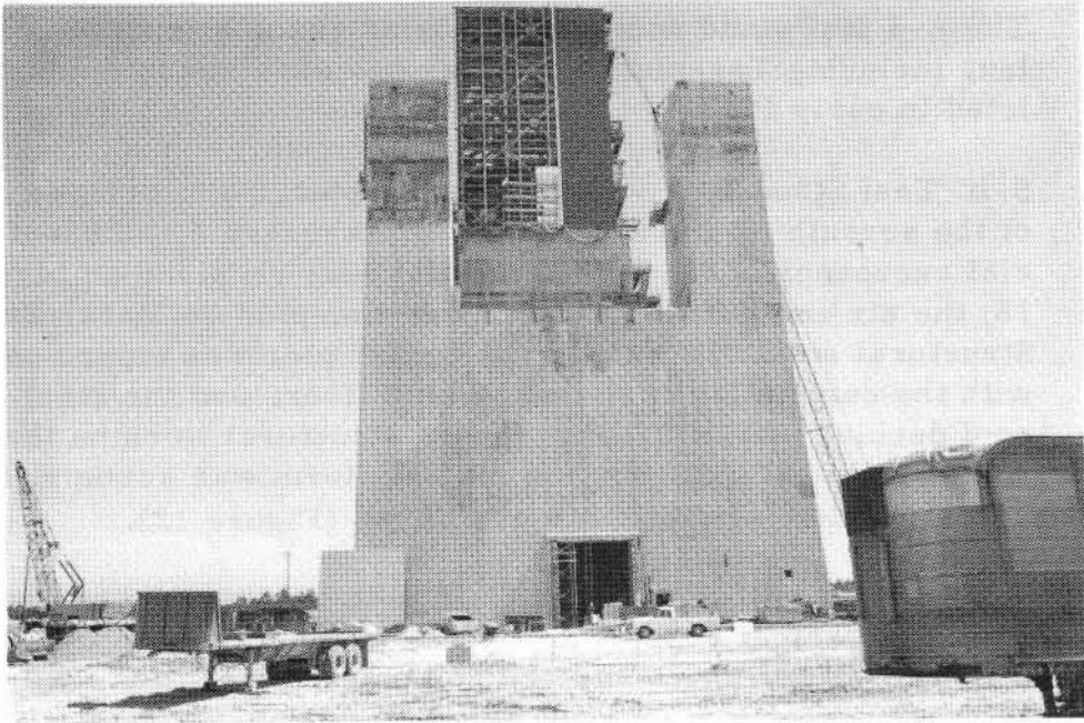
Figure 12 - S-IC Test Stand, West Pier, MTF
