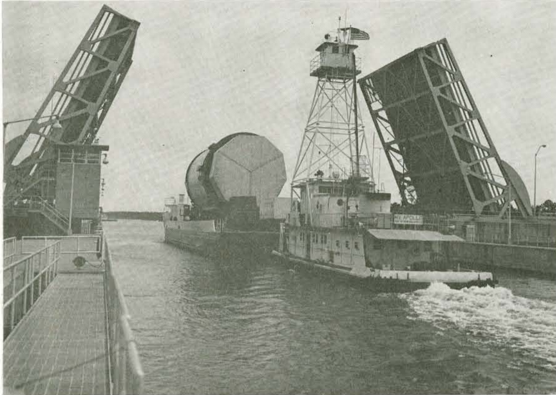
MISSISSIPPI TRAVELER — Bascule Bridge at NASA's Mississippi Test Facility is opened to permit passage of S-II-7, after the stage's 4,000-mile journey from Seal Beach. S-II-7 is due for static test firing at MTF in January, for shipment to Cape Kennedy in March. S-II-5 is scheduled for shipment to the Cape tomorrow; S-II-6 is scheduled to be shipped to KSC Jan. 24.
