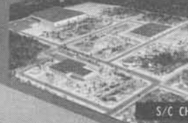
S/C CHECKOUT AREA
