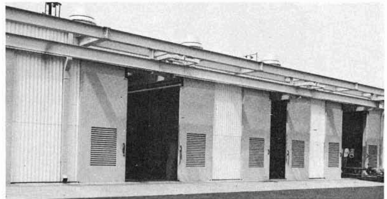
HIGH PRESSURE TEST FACILITY
