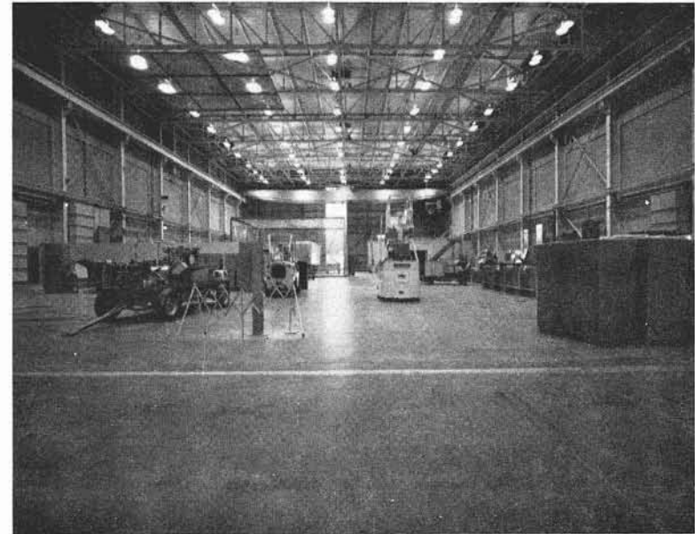
HIGH BAY AREA IN VEHICLE INSPECTION HANGAR
