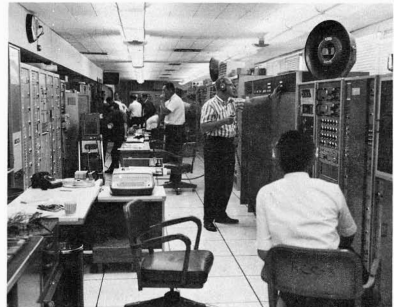
DATA REDUCTION COMPLEX (ANALOG TO DIGITAL STATION IN FOREGROUND)
