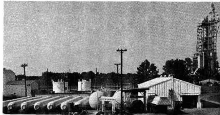
HELIUM BOOSTER STATION
