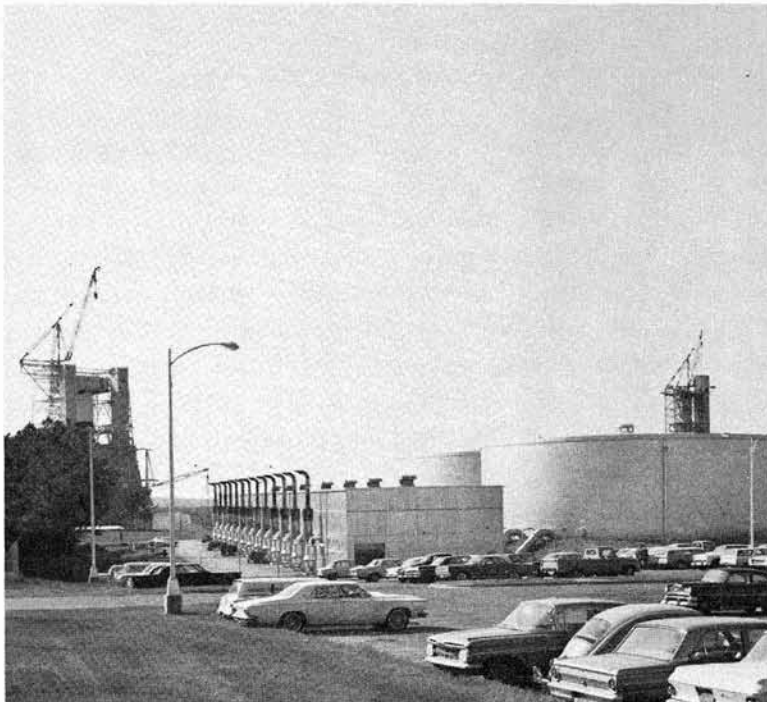
WEST TEST AREA INDUSTRIAL WATER STATION
