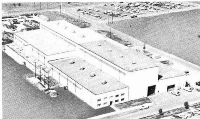
TEST SUPPORT SHOP
