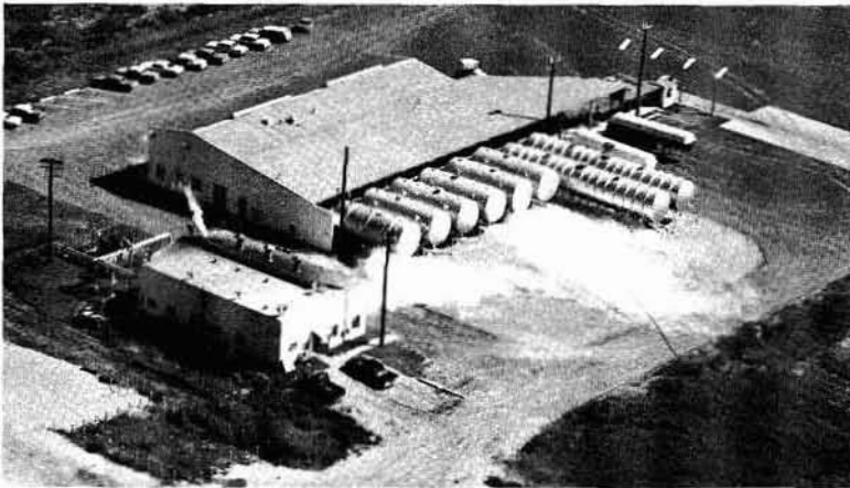
GASEOUS NITROGEN GENERATION FACILITY
