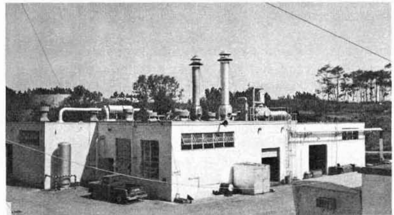
EAST TEST AREA INDUSTRIAL WATER STATION
