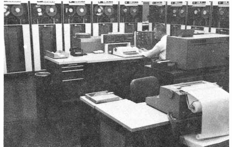
7010 WITH 1050 TELEPROCESSING STATION
