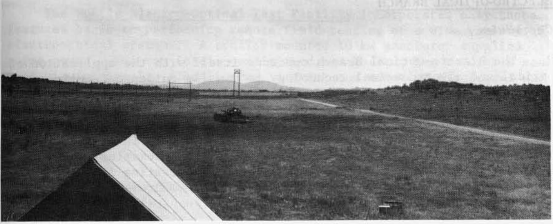
Radar Test Bed Facility
