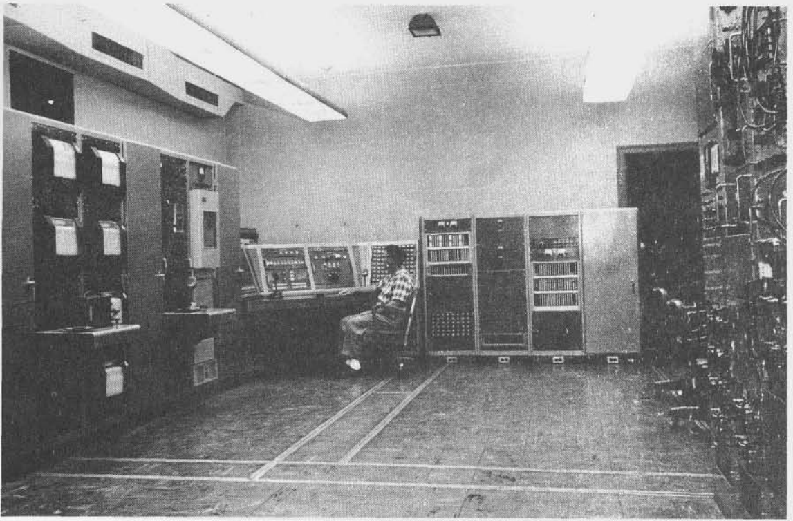
Interior of Instrument Control Building
