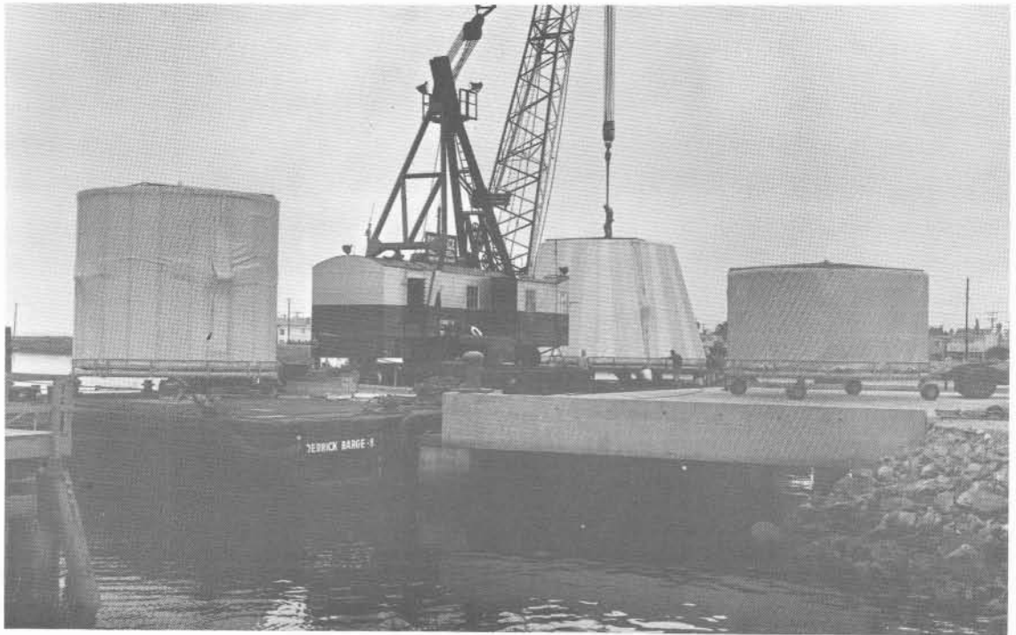
Figure 11. Interstage and Skirt Sections
