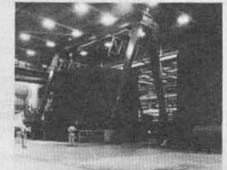
"B" FRAME MOVING SATURN V THRUST SEGMENT
