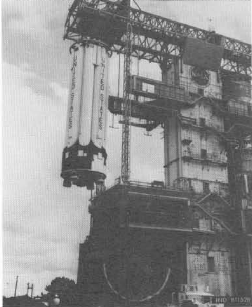
S-IB STAGE ERECTION IN TEST STAND—HUNTSVILLE
