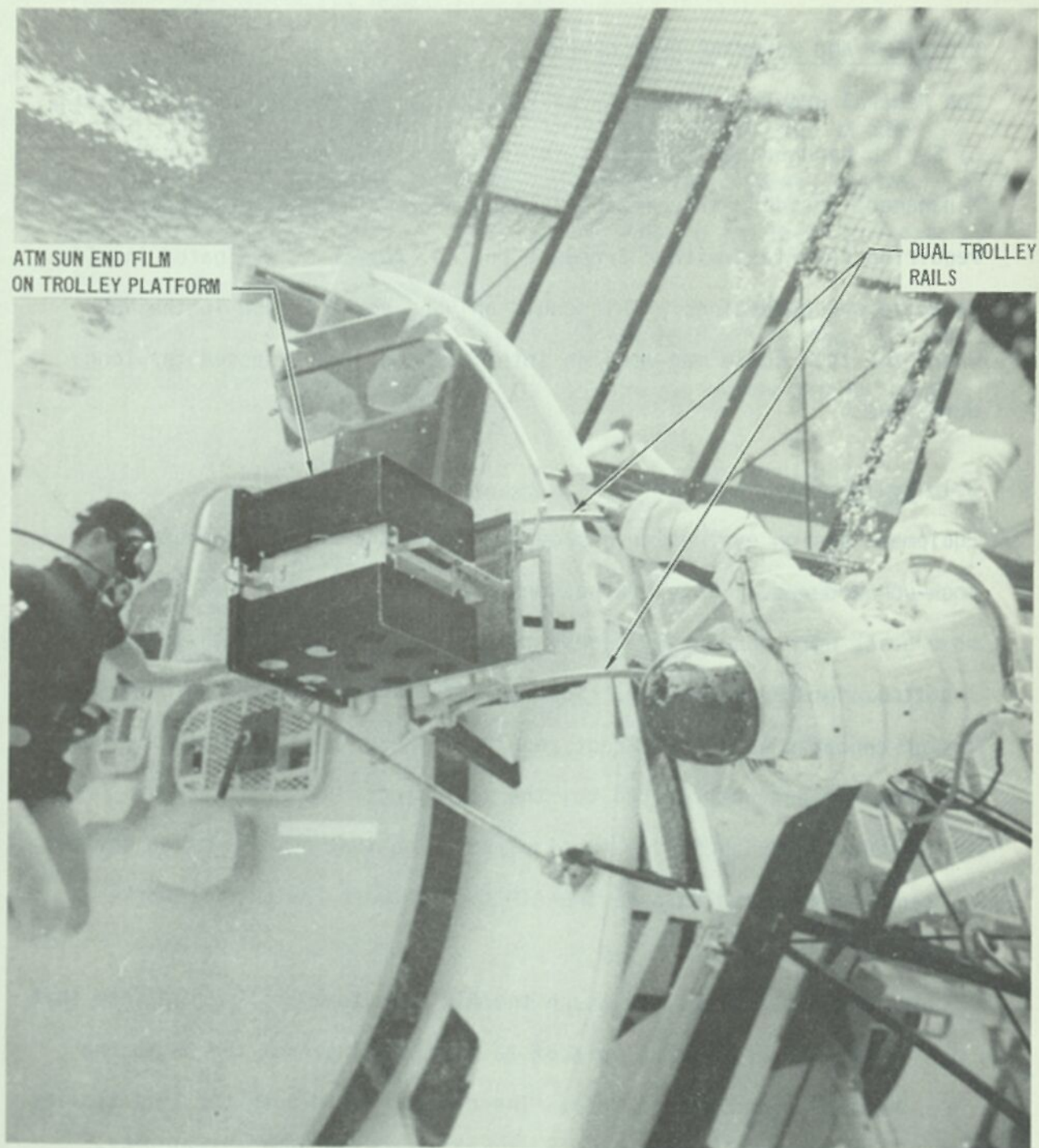
FIGURE 2-1 TRANSLATION OF ATM FILM TO SUN END WORKSTATION USING PRELIMINARY "TROLLEY" CONCEPT
