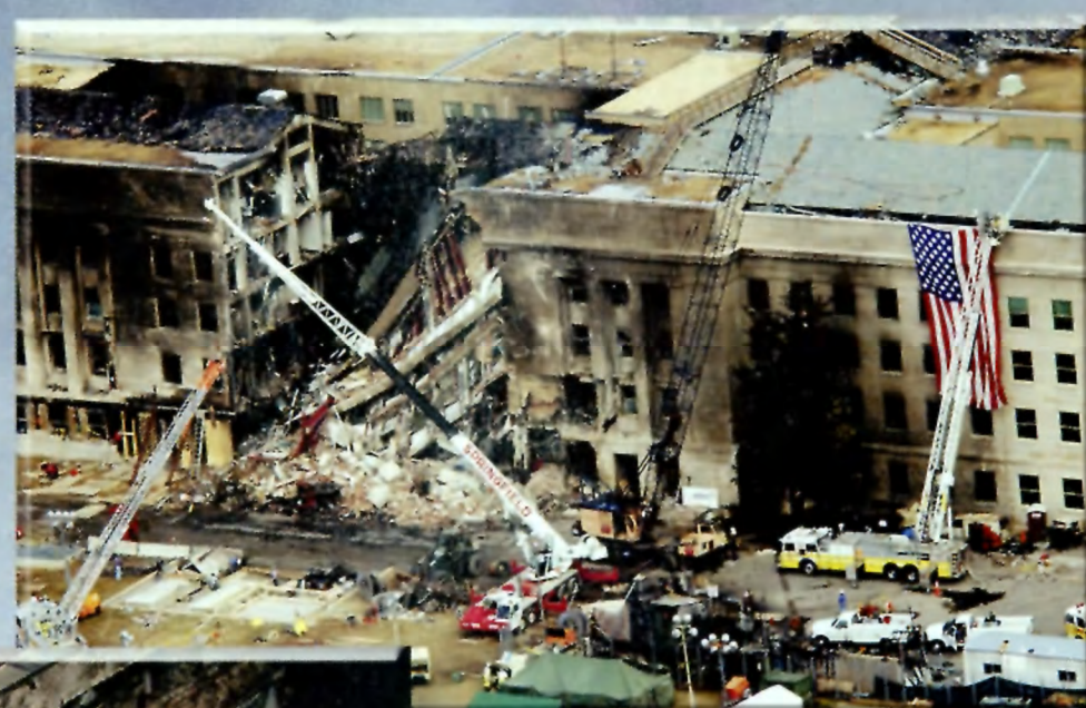
Collapsed portion of Wedge One showing the blast-resistant windows and steel frames still in place. Fire damaged the wooden roof and limestone facade. Replacement limestone will come from the same quarry in Indiana as the original stone.
