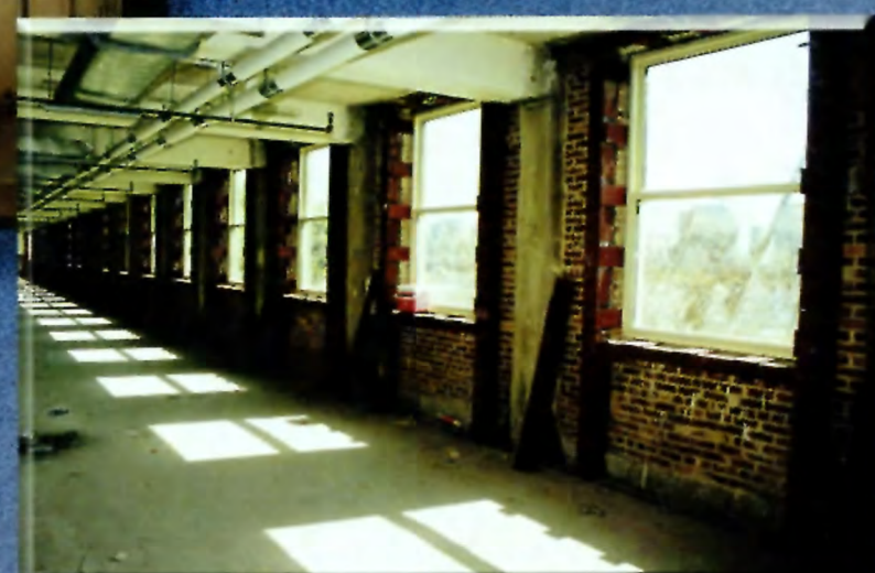
New blast-resistant windows were installed but maintained historic features such as handles, screen holders, and sashes. Steel beams supported the weight of the new windows while a Geotech panel, to prevent fragmentation, covered the original brick and mortar.
