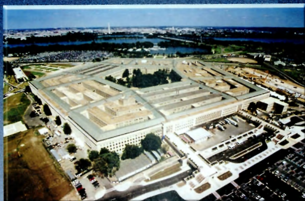
A completed Wedge One (lower left of picture) with historic facade on September 5, 2001.
