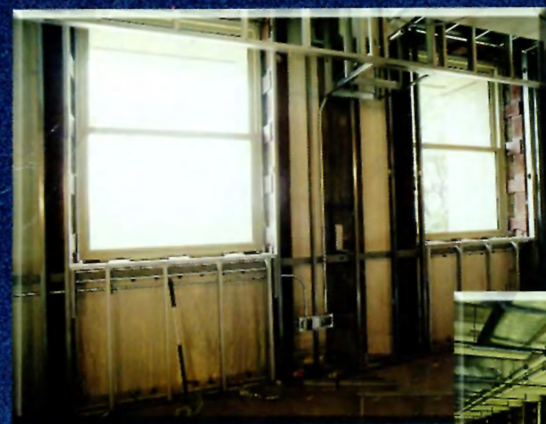
New blast-resistant windows were installed but maintained historic features such as handles, screen holders, and sashes. Steel beams supported the weight of the new windows while a Geotech panel, to prevent fragmentation, covered the original brick and mortar.
