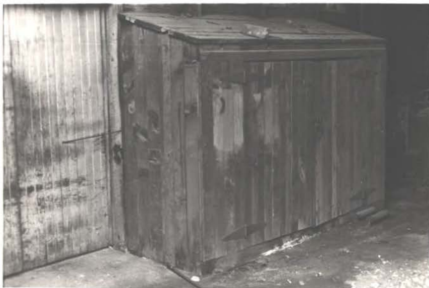
STORAGE SHED (INTERIOR) →
