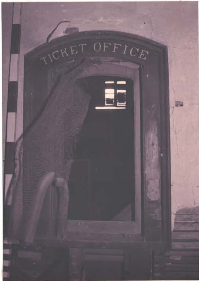
bH (10) N. Corridor beyond (view in hall)
