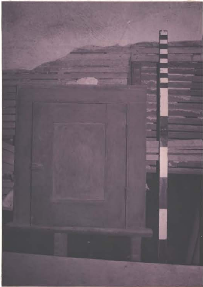
bH (8) door to hall from N. Corridor
