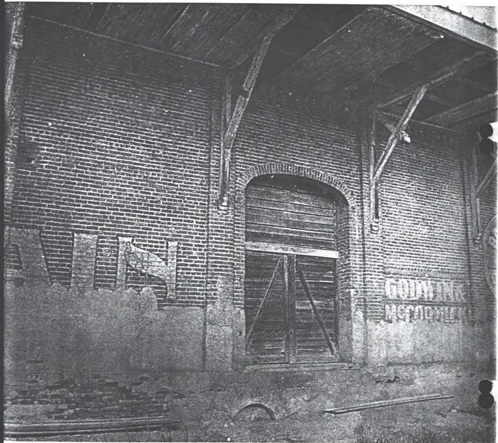
Vicksburg and Brunswick Depot. Detail of storage area door and advertisements painted on walls.
