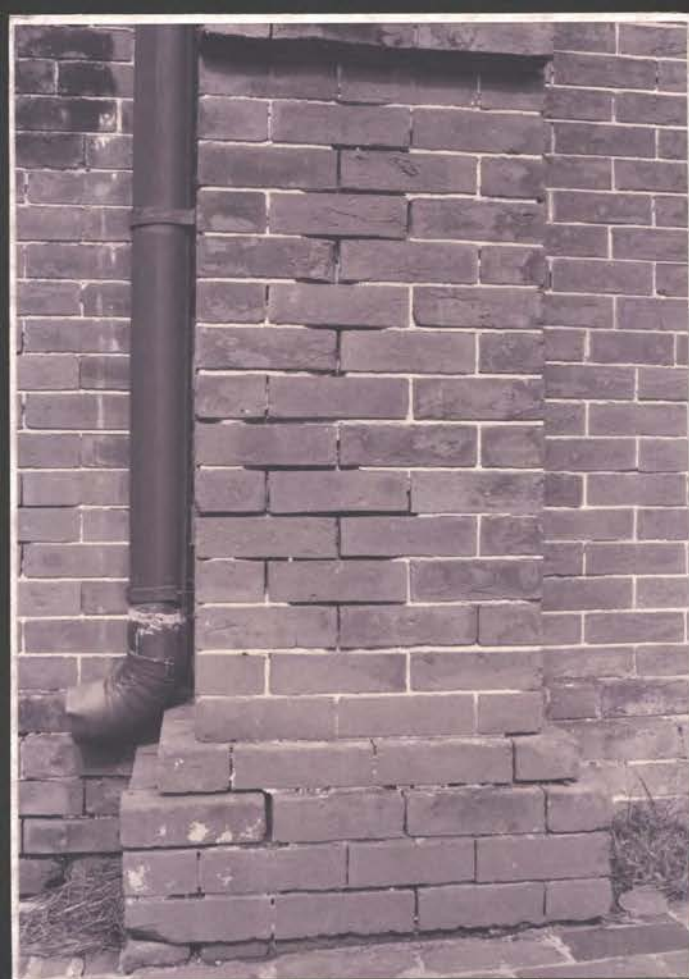
DOWNSPOUT DISCHARGES DIRECTLY ON BRICK, JTS. ERODED (N. OF N.W. ENTRY)
