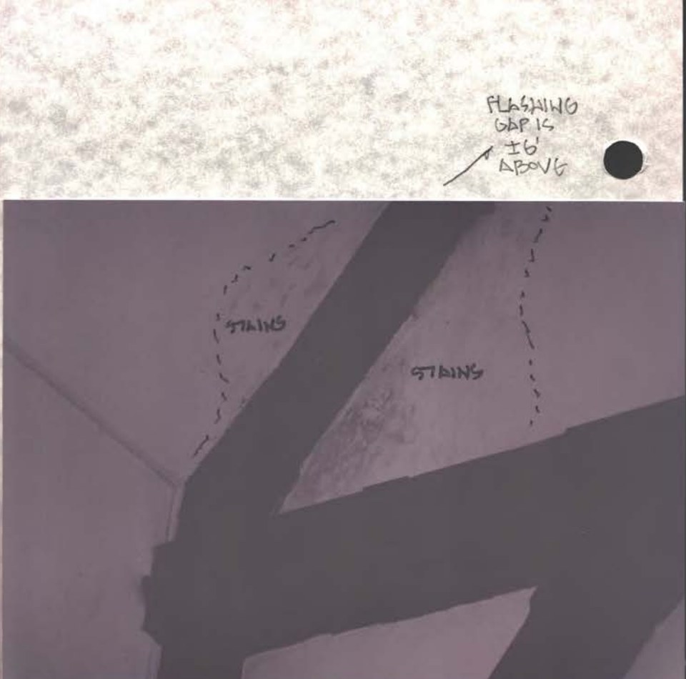
S.W. CORNER AT TOWER SEE P. 10 PHOTOS
