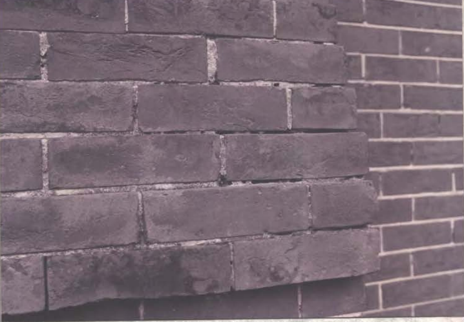
ERODED JTS.
