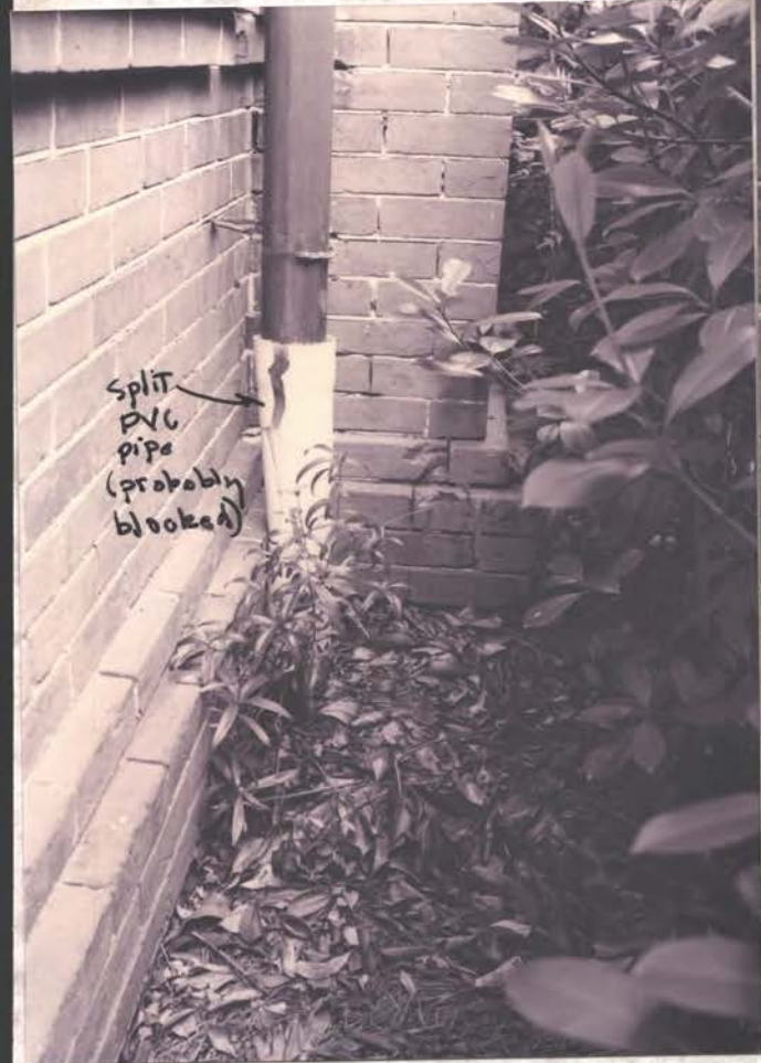
DOWNSPOUT DISCHARGES DIRECTLY ON BRICK, JTS. ERODED (N. OF N.W. ENTRY)
