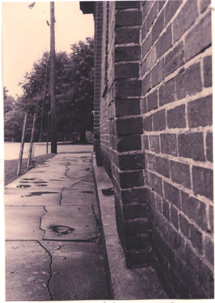
Rt. Corner at St. intersection (combined rising damp + footing rotation)
