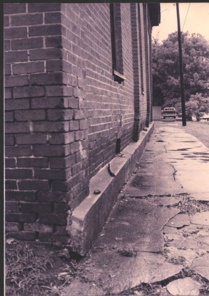
Rt. Corner at St. intersection (combined rising damp + footing rotation)
