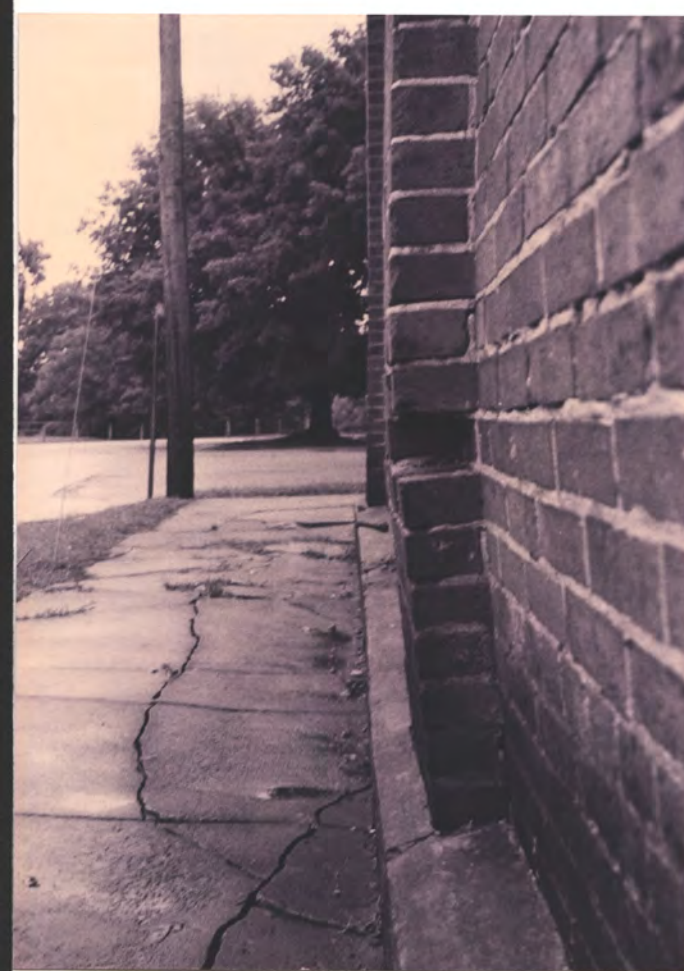
2ND PILASTER walk bowed due to foot. rotation
