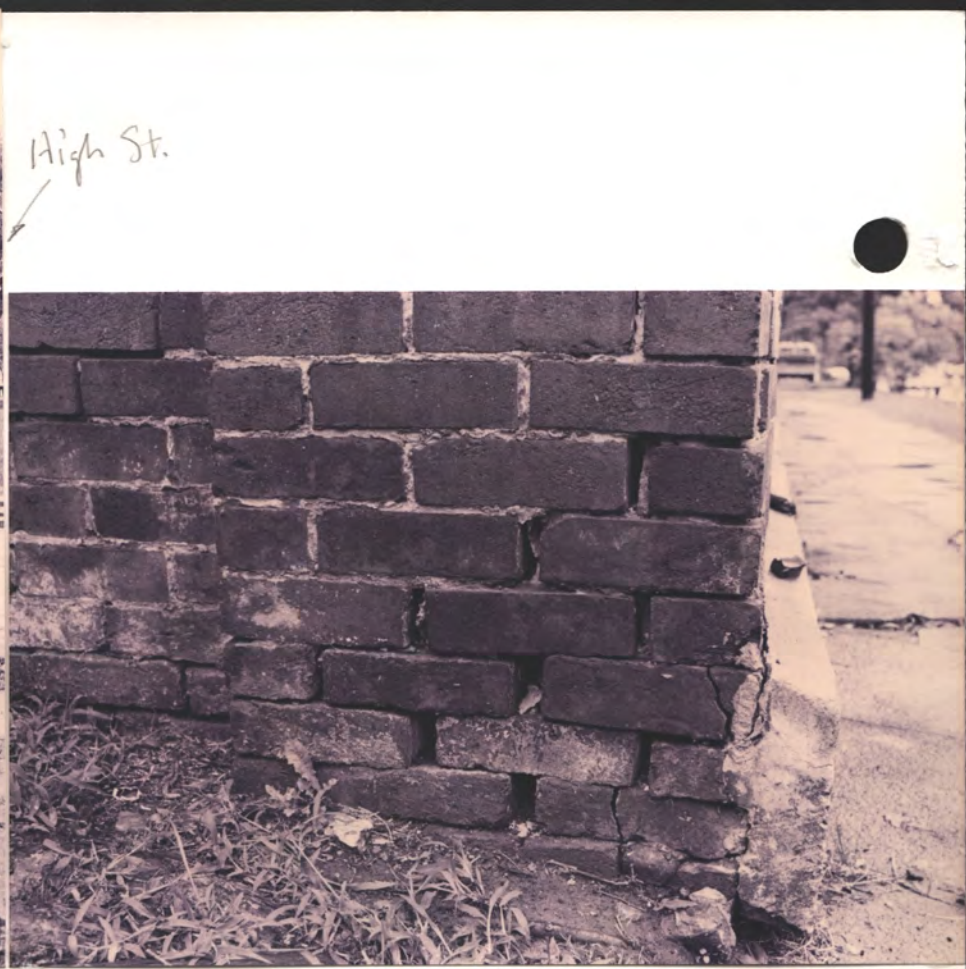
Rt. Corner at St. intersection (combined rising damp + footing rotation)
