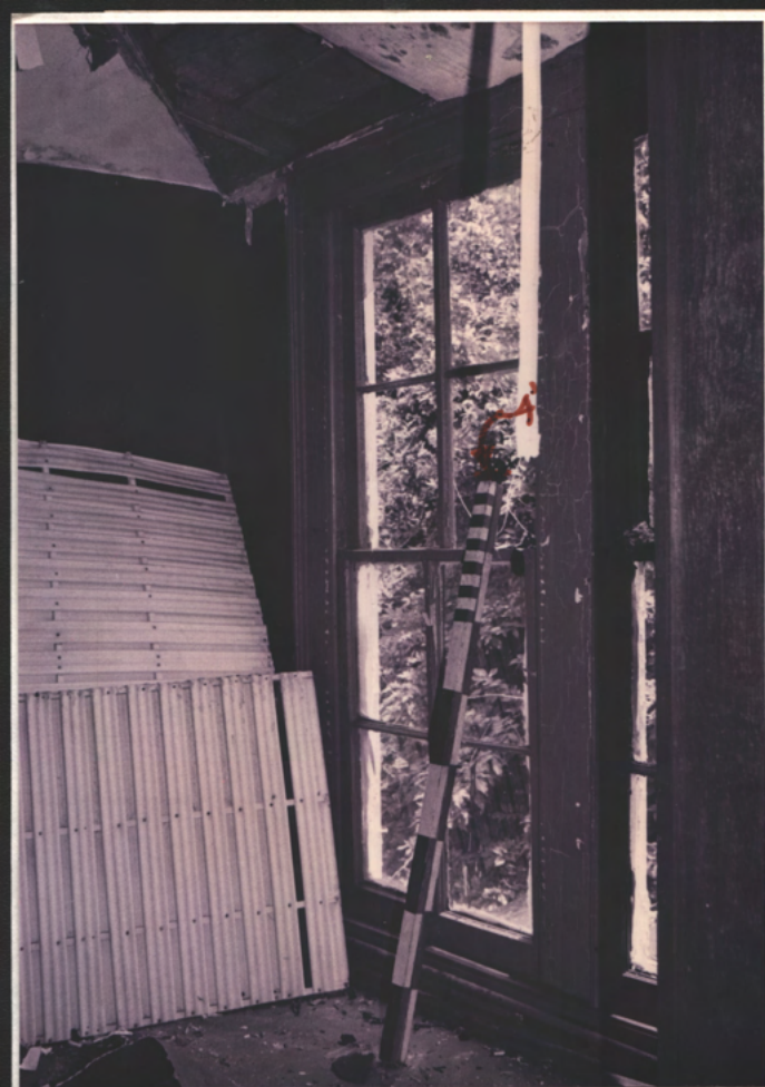
Enclos. S. Porch Run just east of S.W. End Run, Et. 2
