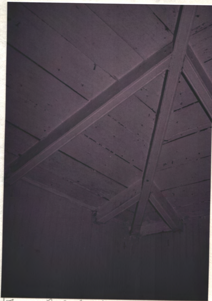
Roof at S.E. corner (Vic. banded joints/rafters)
