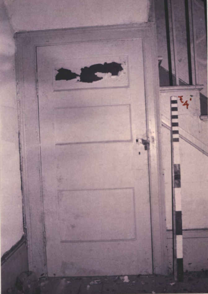
→ Door to orig. chas. under W. front stairs. 3-horiz. panel is c. 1838 (junk-plank marks etc) = removed for 1838
