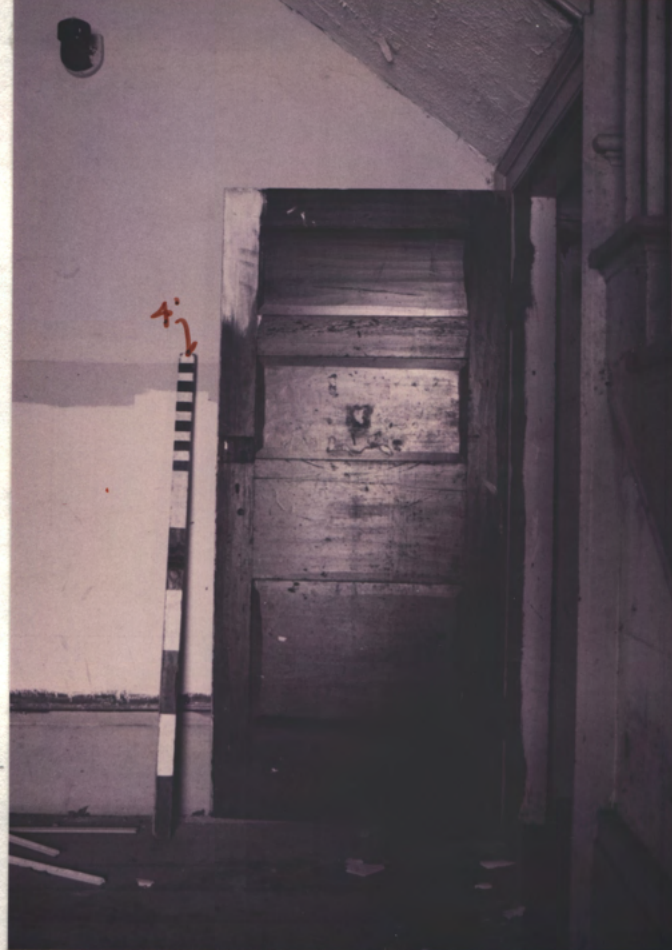
→ Door to orig. chas. under W. front stairs. 3-horiz. panel is c. 1838 (junk-plank marks etc) = removed for 1838
