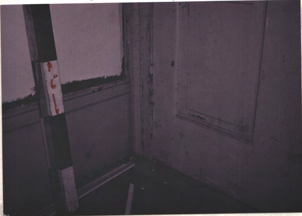
E. Door of W. Gallery, to E. Central Room (E. side, or early) Cast iron one-pc. ("fast-pin") early hinge.
