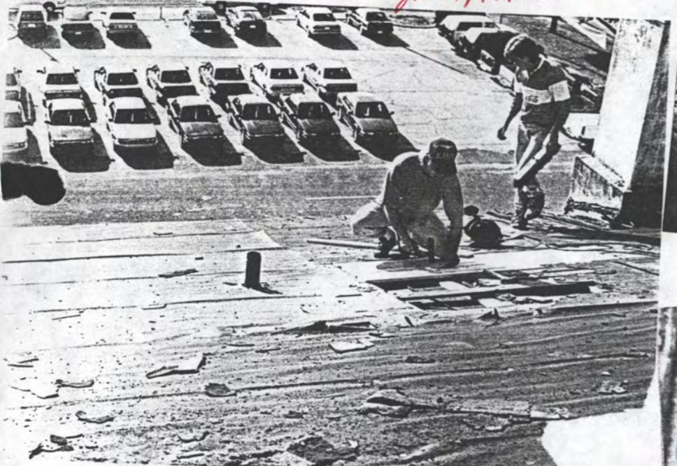
photo shows the "double decking with fascia boards removed
