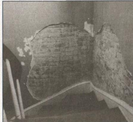
↑ MORE THAN 600,000 BRICKS WERE ORDERED FOR THE CONSTRUCTION OF THIS HOUSE. THE WALLS OF THE HOUSE MAY BE AS MANY AS FOUR LAYERS OF BRICK THICK TO INCREASE THE HEATING AND COOLING EFFICIENCY OF THE DWELLING. THE BRICKS WERE SURFACED BY MASTER PLASTERERS BOTH INSIDE AND OUT.
