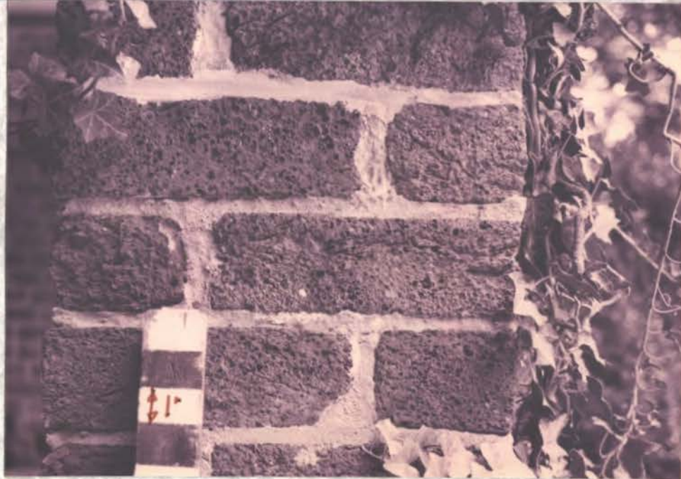
HEAVY sandblasted brick prior at lower part of portico
