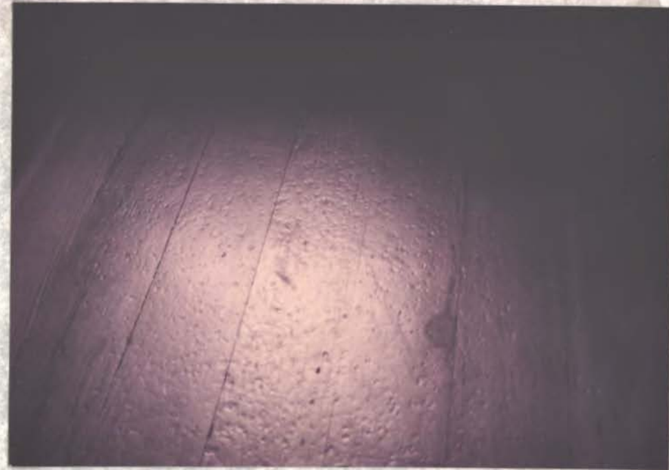
spike-heel dents (fl. was sanded in 1980's per the mus. mgr.) PN
