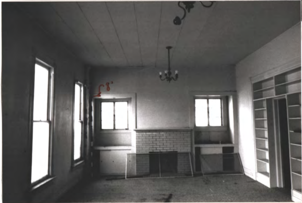
Parlor. = Mod. f.p. f end-windows gypsum bd. on all walls. mod. Shelves
