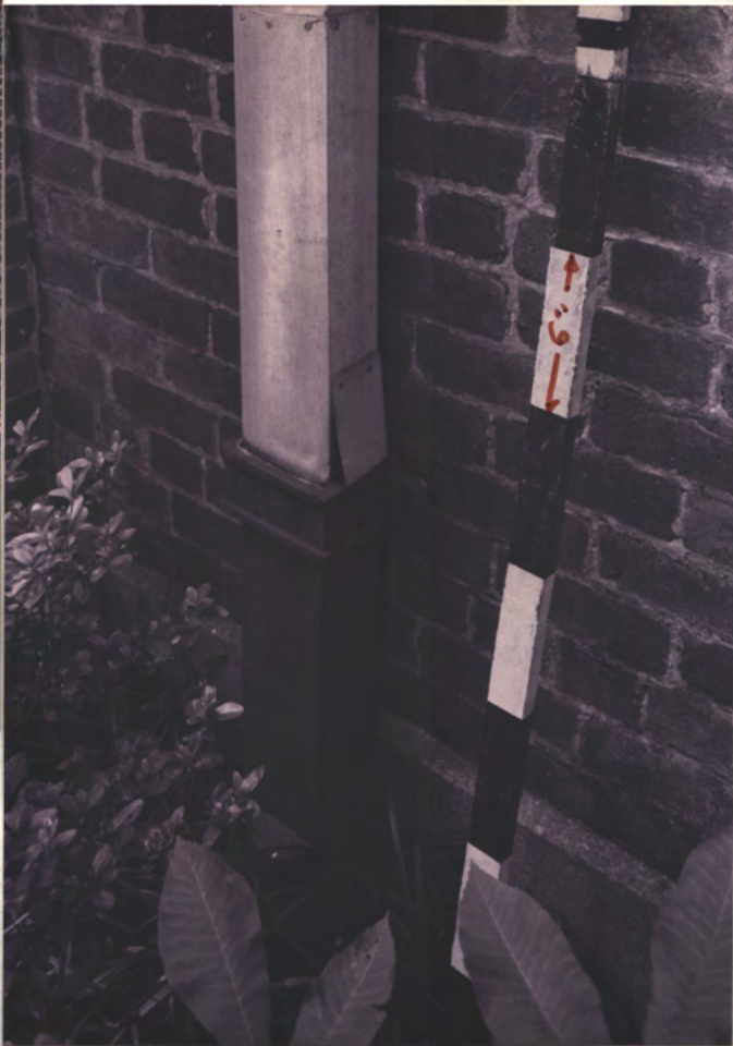
Downspout at left photo, puffed - not split.
