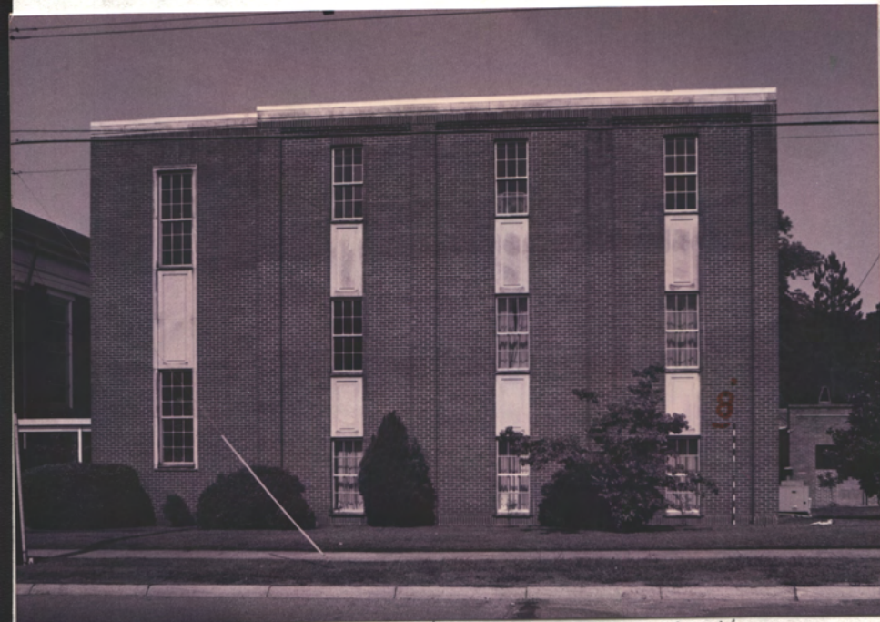
① → East front of 1950's N. Wing (Fellowship Hall) at FL1, CRs at FL2
