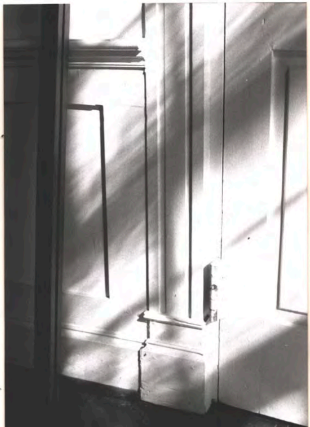
1830 east door, hinges & "Carpenter" lock
