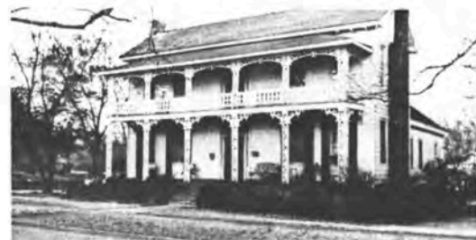
THE PETERS HOME, ca. 1860, displays beautiful saw work by master carpenters. West DeKalb Street.
