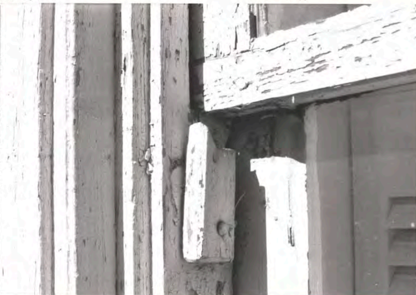
20th. c. stucco (Portland) see c. 1860 photo - no stucco 1830 sashes (pegged) → holdopen for lower sash (typical of Fed. period except usually inside) mod. →
