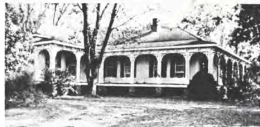
THE COCKE-GIBLER HOME, ca. 1830, is outstanding for its ceiling medallions and frieze work. Highway 45.
