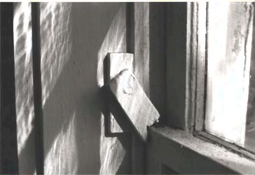
Sash locks (typ. Fed. type) 1st fl., 2 diff. loc. shown
