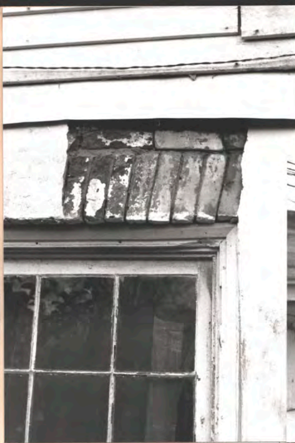
Jack-arch, 1st fl. east (typical) → N Stucco = mod. com
