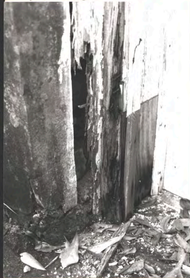
Note unmet brick jamb, mura that opens to orig. → N
