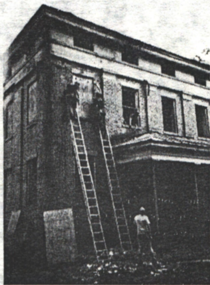
Clanton Boy Scouts, under the leadership of Kirk Stokes, and members of the Elm Bluff Hunt Club helped stabilize the Greek Revival-style house by boarding windows and clearing the grounds.
