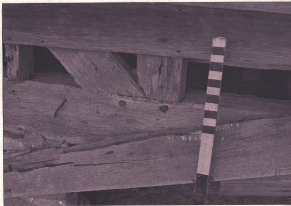
↑ Note pegs at mortise of tenon joints (typ. of 1800-1870±)
