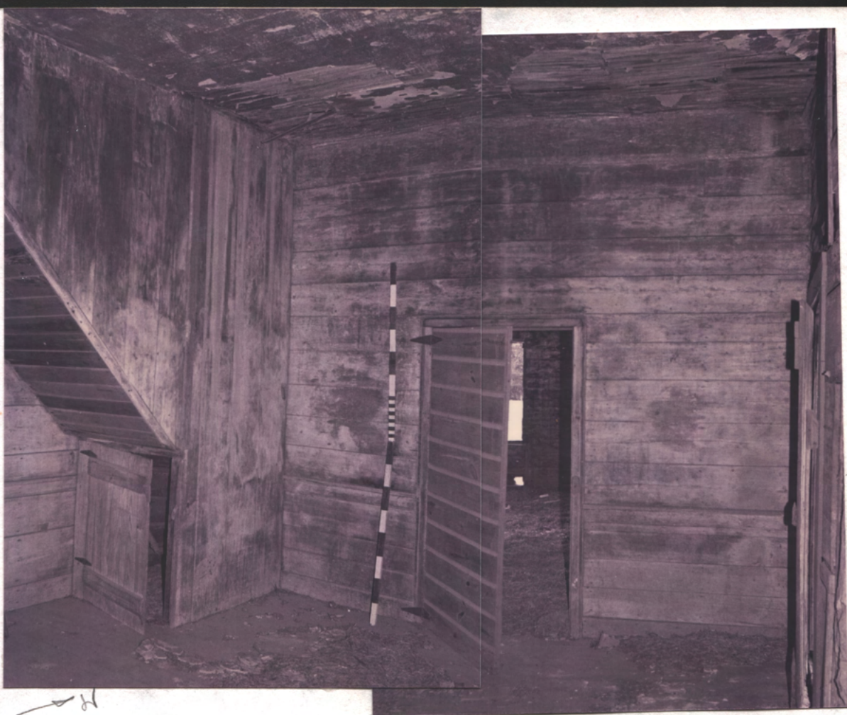
N. WALL of S.E. RM ← modern door in orig. frame
