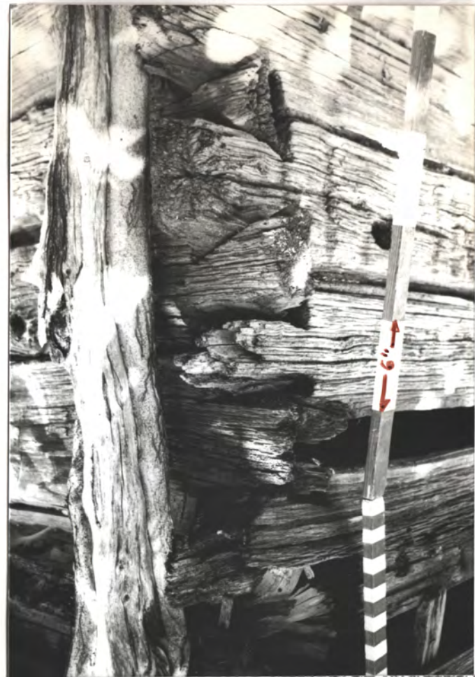
Smoky Mts, c. 1835? SE. Corner FULL DOVETAIL JOINT (MOST VISIBLE)
