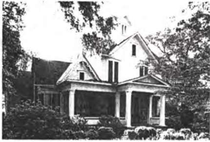
OAKSIDE ca 1873 • Chilton County
