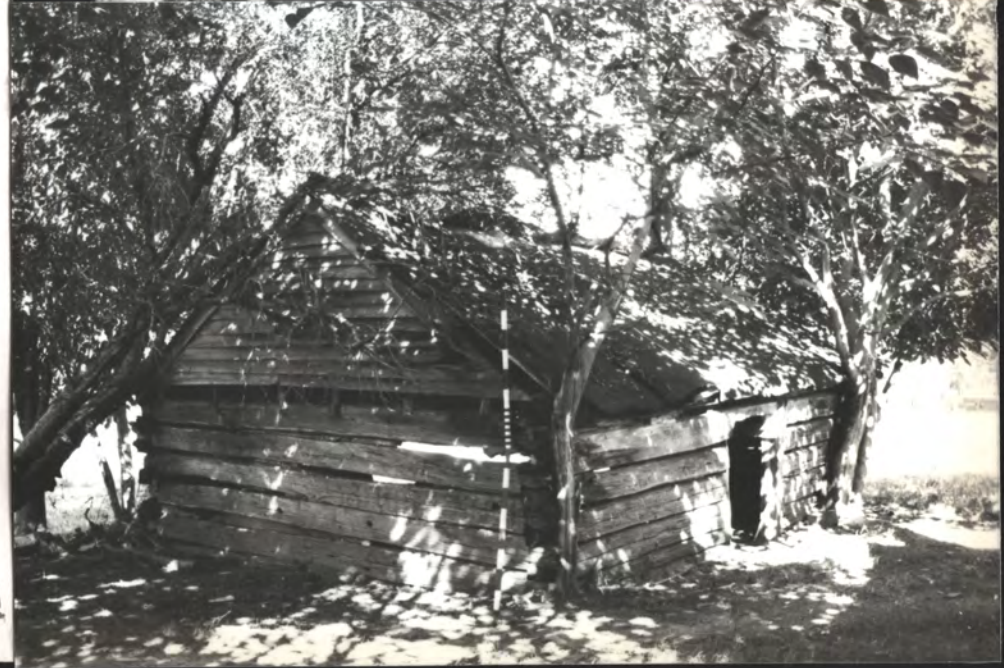
Smoky Mts, c. 1835? SE. Corner FULL DOVETAIL JOINT (MOST VISIBLE)
