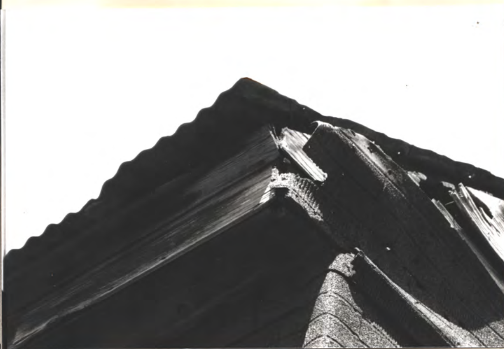
S.W. Corner Main Roof
