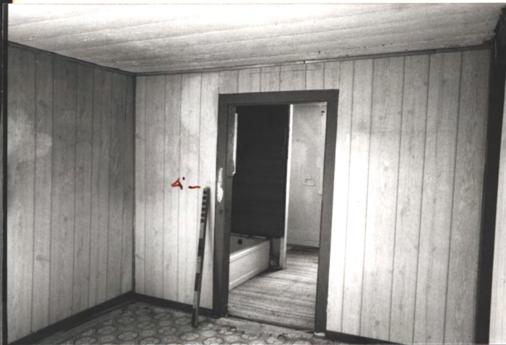
1st fl. West central rm. probably open porch originally (verify)
