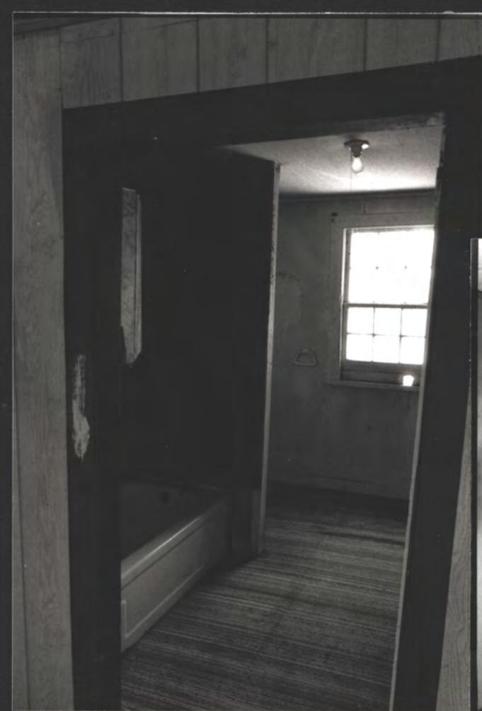
1st fl. N.W. Shed Rm
