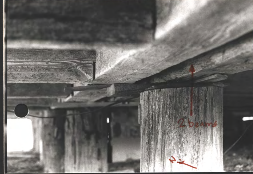
Note apparent "addition jt." between front + rear shed →
