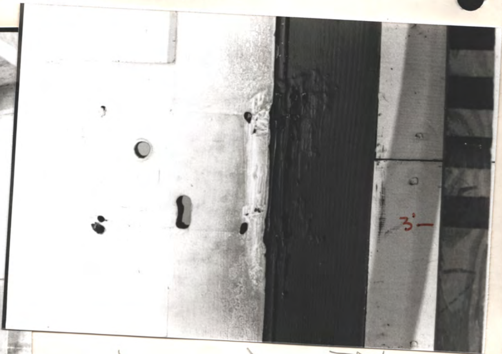
1st fl. N. Rm., east door to rear porch
