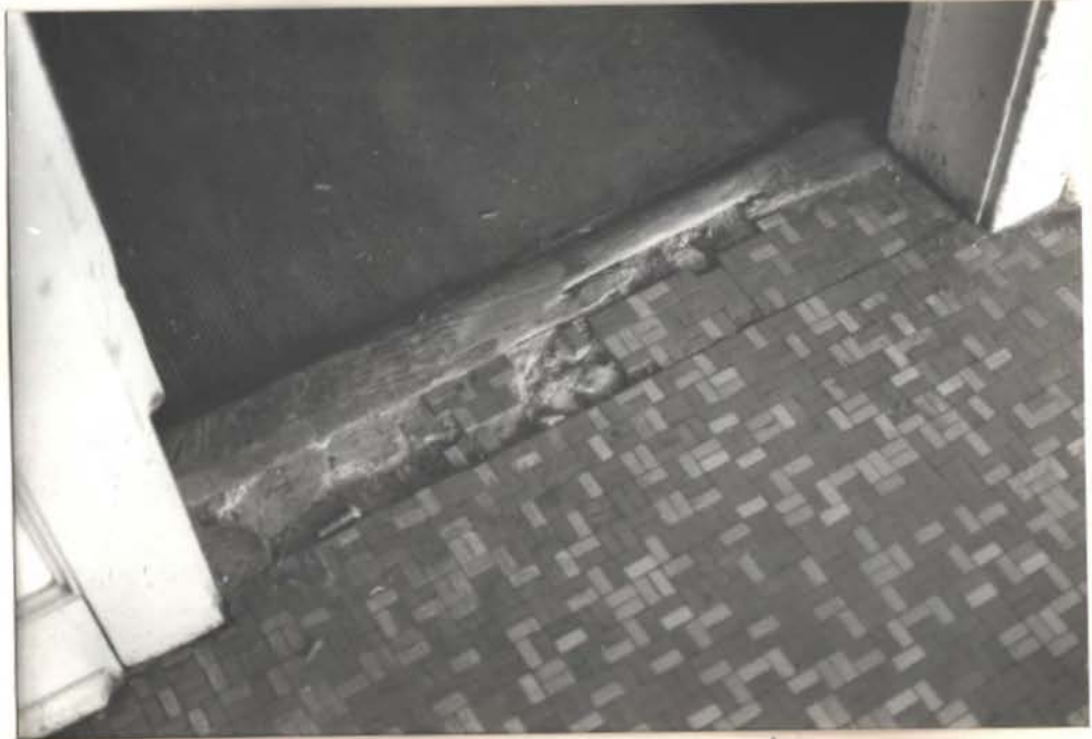
Door from lobby into 1st fl. Guest lin hall
