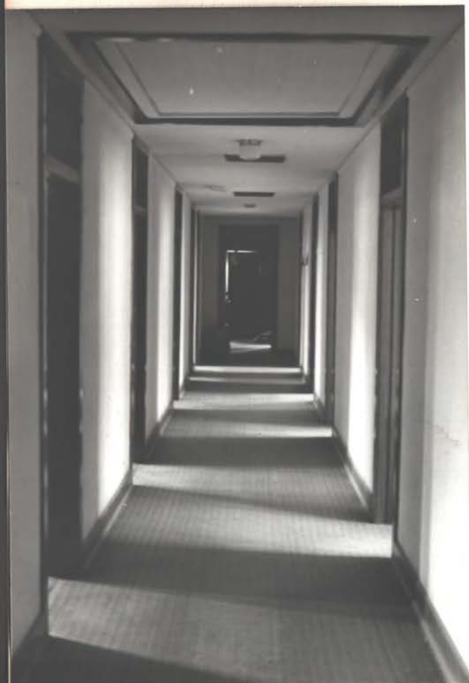
2nd fl. main hall → N (Ceil. rect. = exhaust fan? Skylit?) ↑ N
