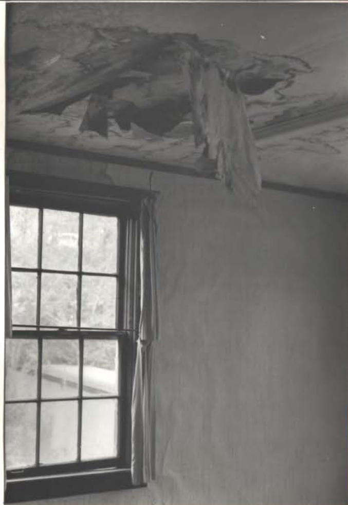
N.W. 2nd fl. rm. in attic.
